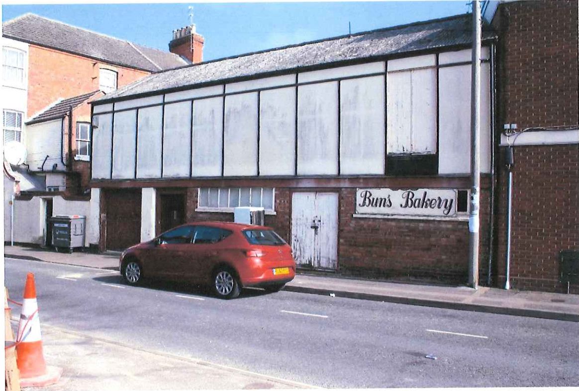
View of existing building from Victoria Street
