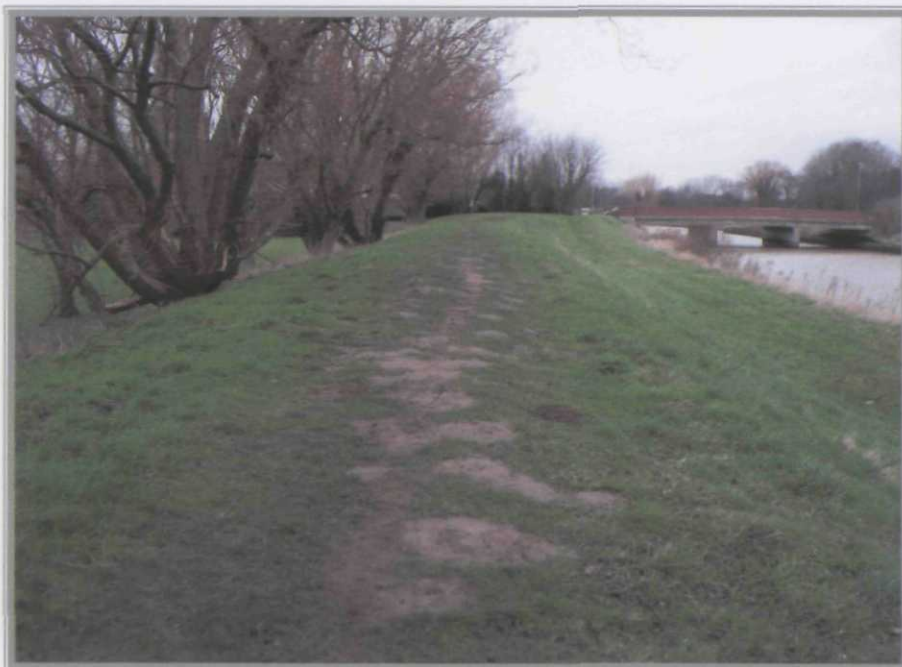
Coronation Channel Embankment – U.S. from A151 Bridge
