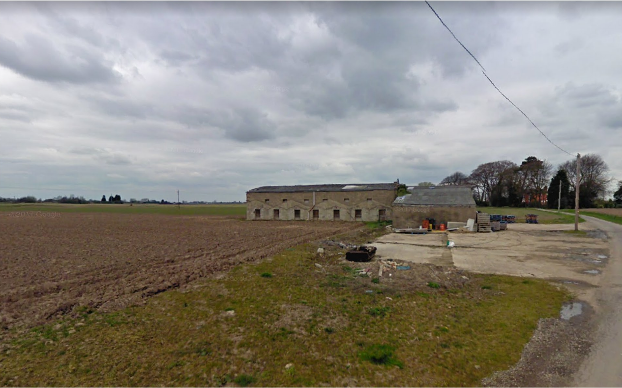
South East Elevation seen from Scoldhall Lane. From the differences in block colouration (forming a gable shape) we can assume the barn was larger at some point.
