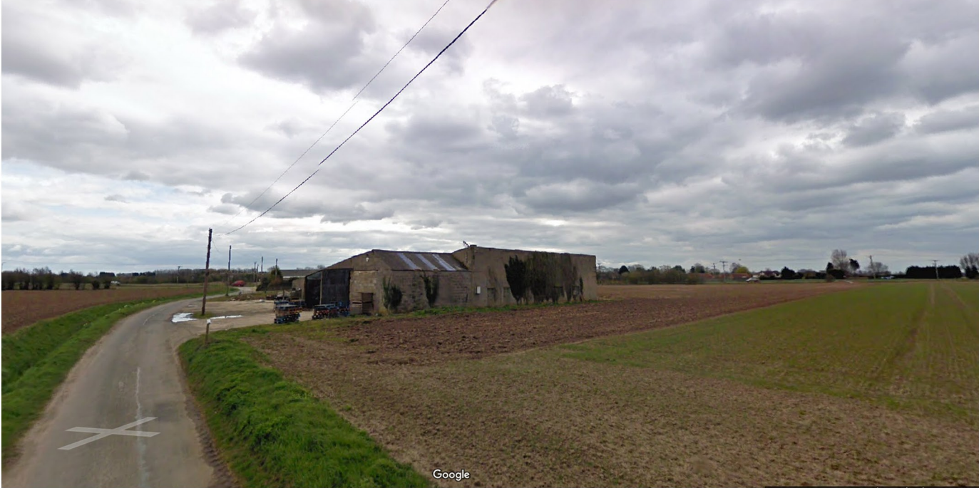
North West elevation seen from Scoldhall Lane.
