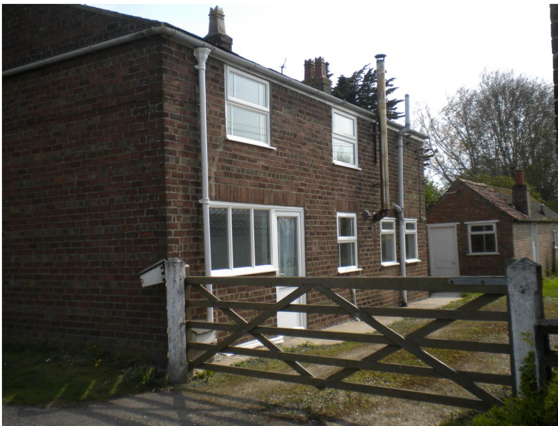
North Elevation showing the Extensions carried out in the Early 20 th Century together with the existing access.
