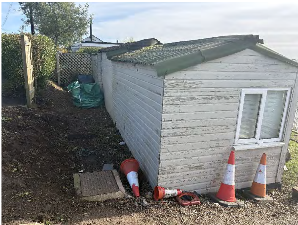
Rear of shed / summer house
