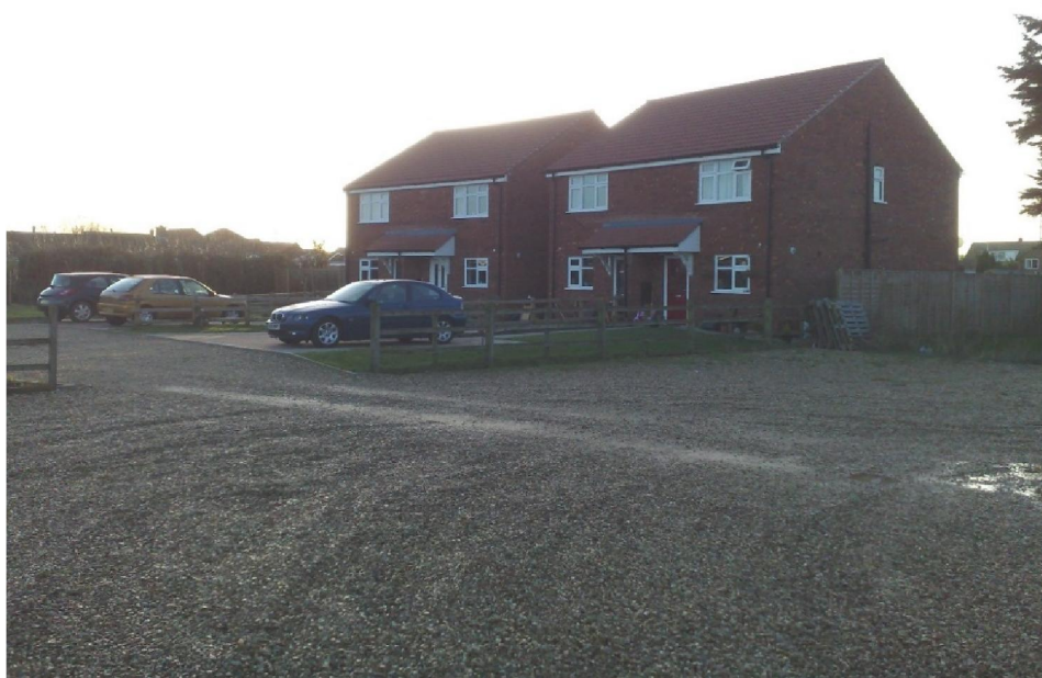
Photo 2: Adjoining South Holland District Council new-build for rent.
