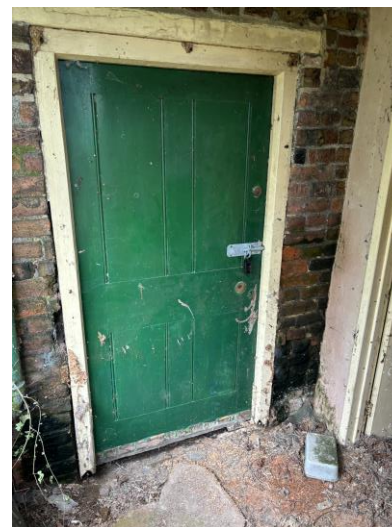
Photograph 2 Measures taken to limit unauthorised access
