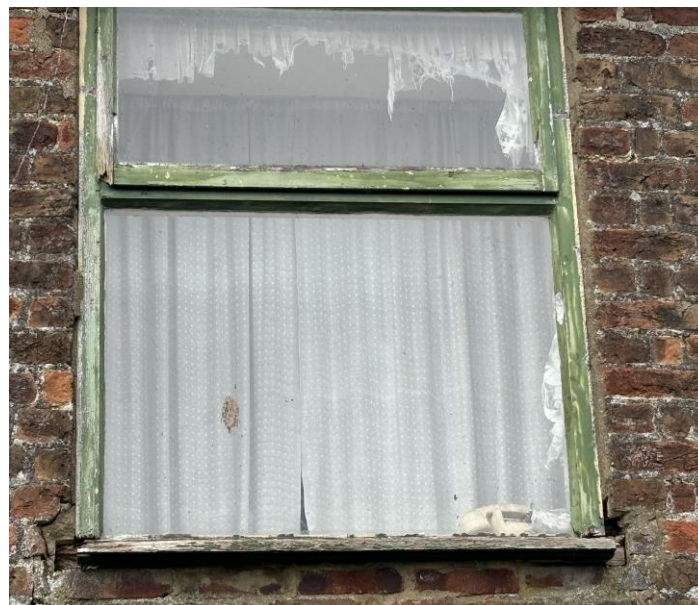
Photograph 5 Close up of a Window showing secure glazing and curtains
