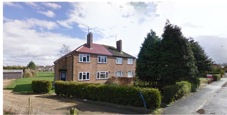
Image 10 - Showing properties opposite the site
