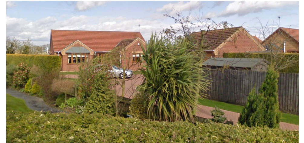
Image 11 - Showing properties opposite the site
