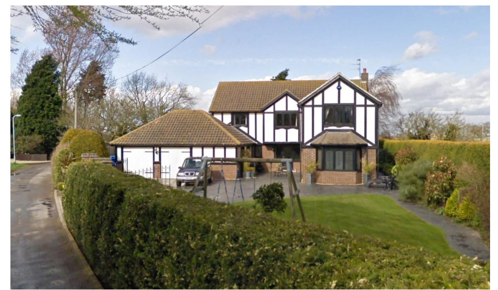
Image 8 - Showing properties opposite the site
