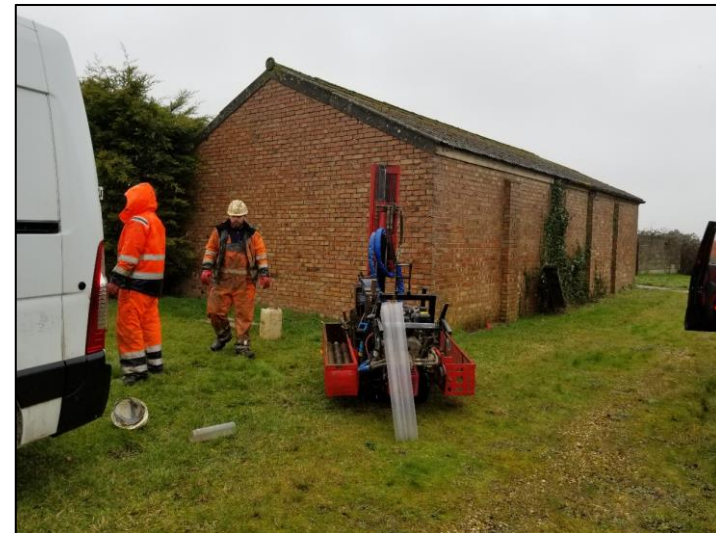
Photo 4 - Southern Storage Building
