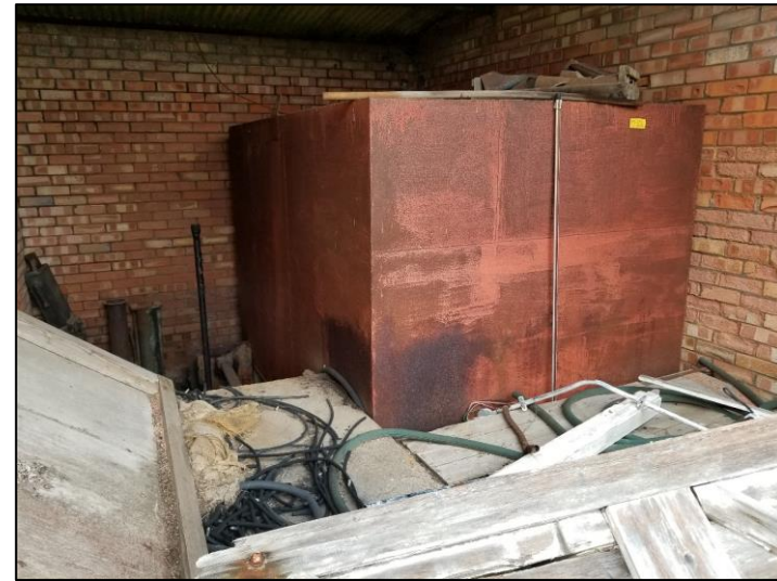
Photo 2 - Above Ground 'Gas Oil' Tank
