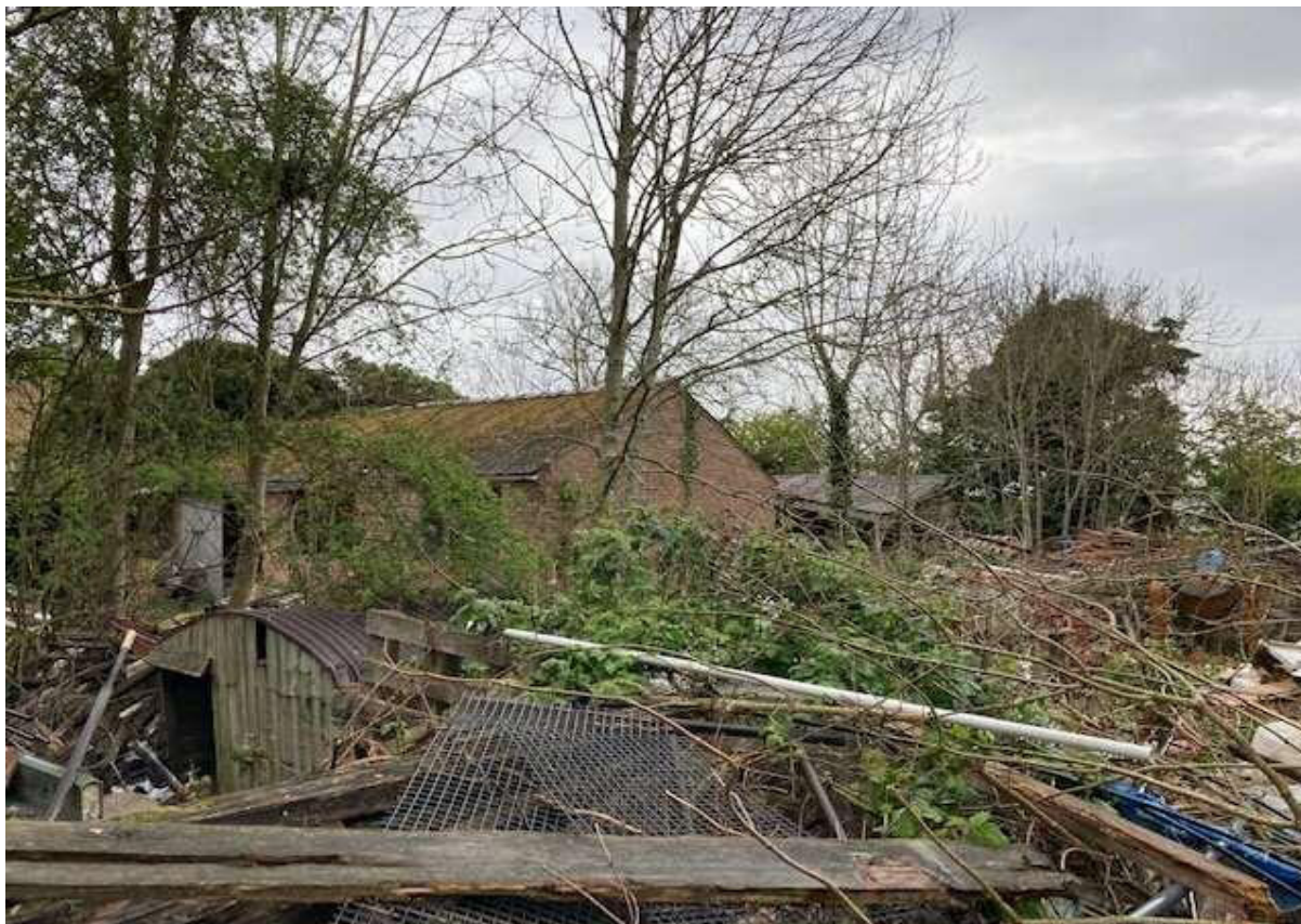
View of existing buildings from east side
