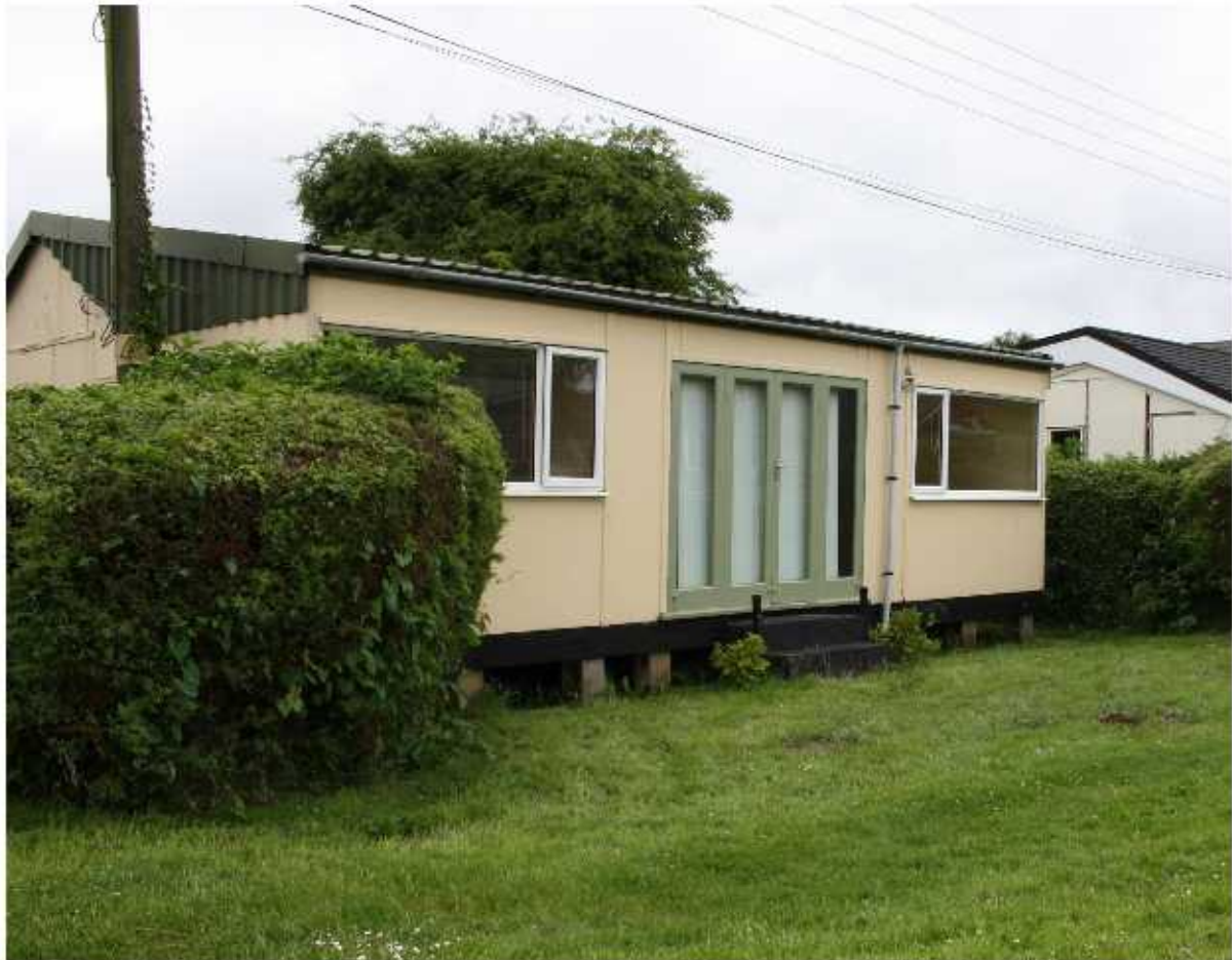
View of existing property from alongside river
