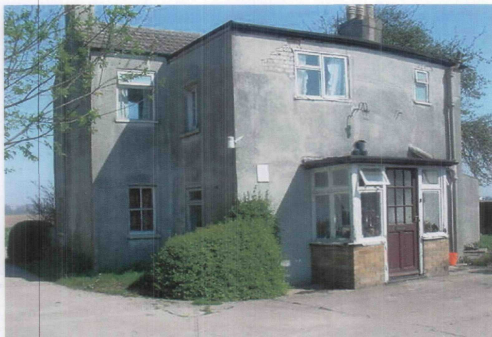
Plate 2; Rear of dwelling
