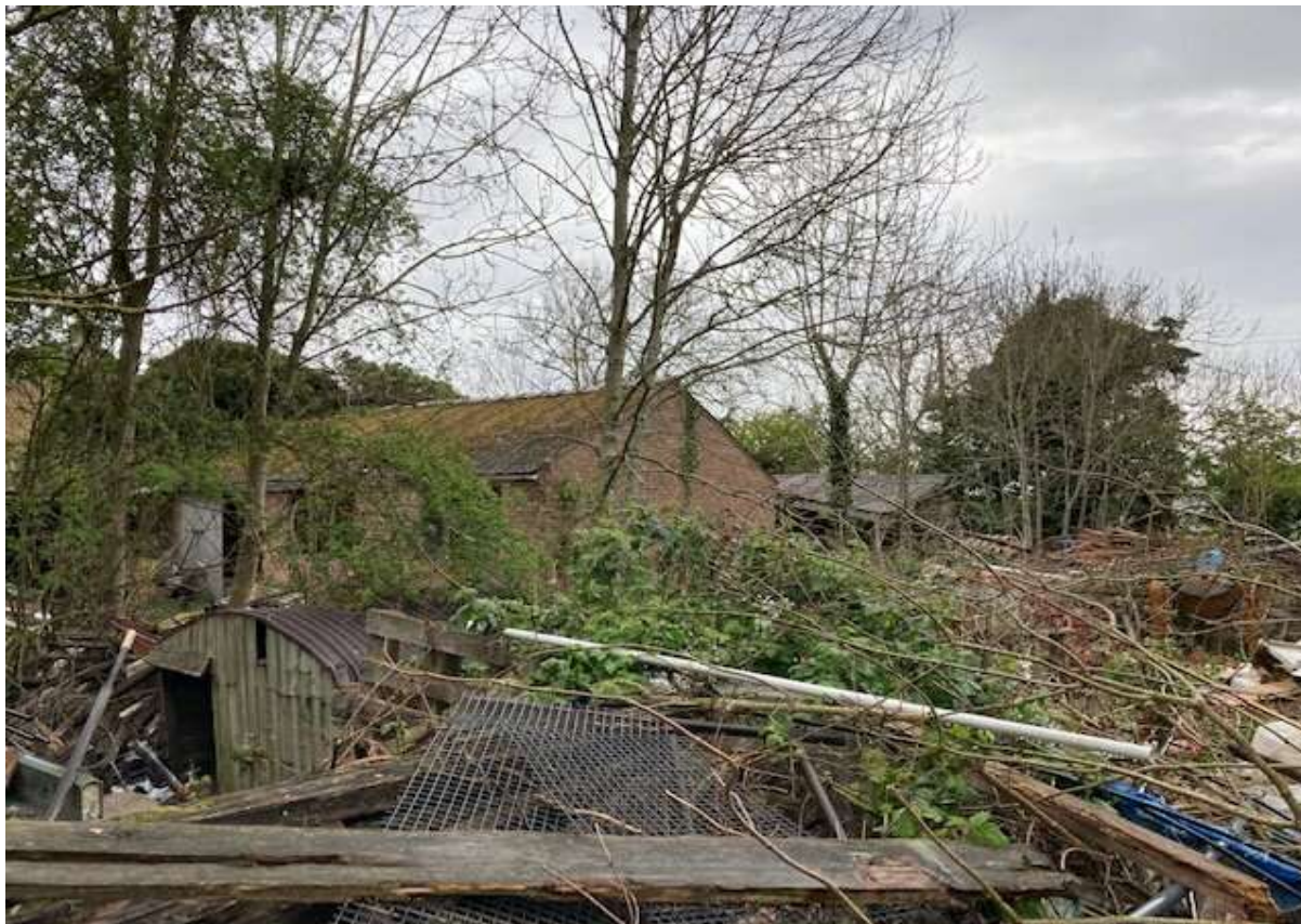
View of existing buildings from east side
