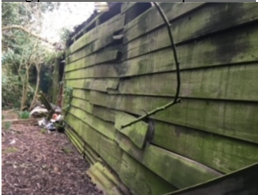
Timber cladding to front wall
