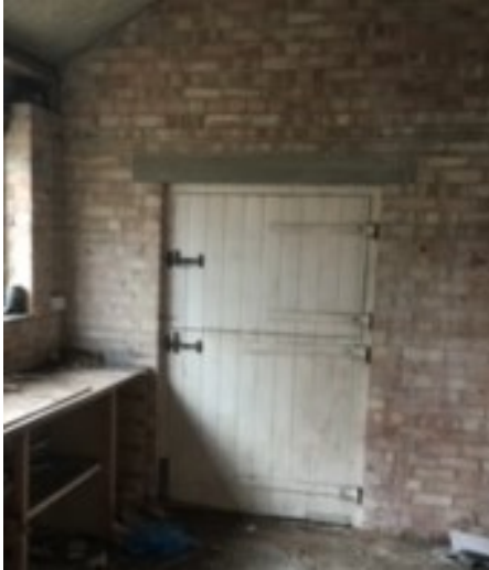
Original stable doors
