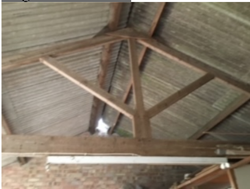
King post trusses in workshop and stores
