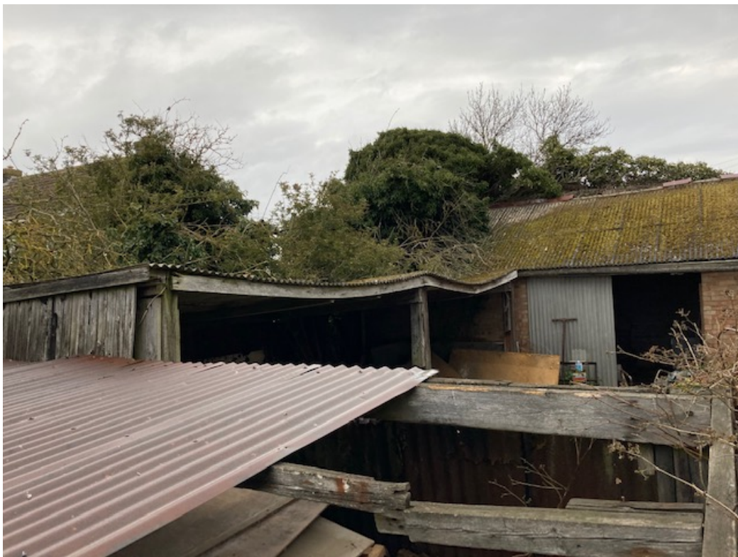
View over potting shed looking back towards main building
