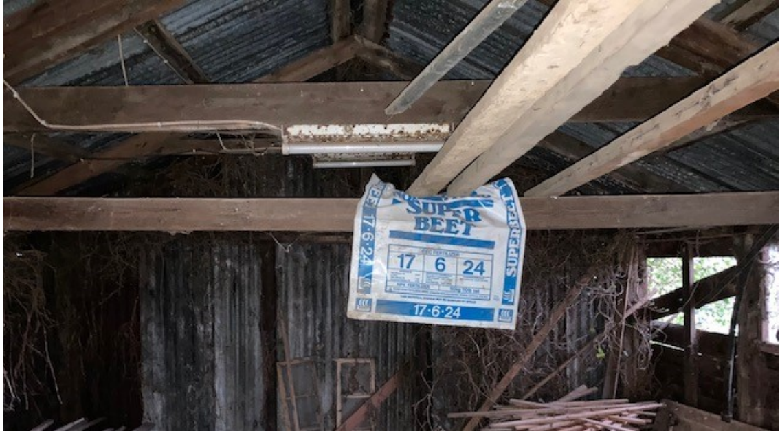
Roof structure in tractor shed
