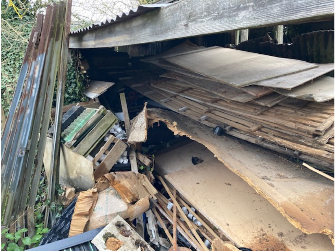
Former pots/seed trays and shelving within potting shed
