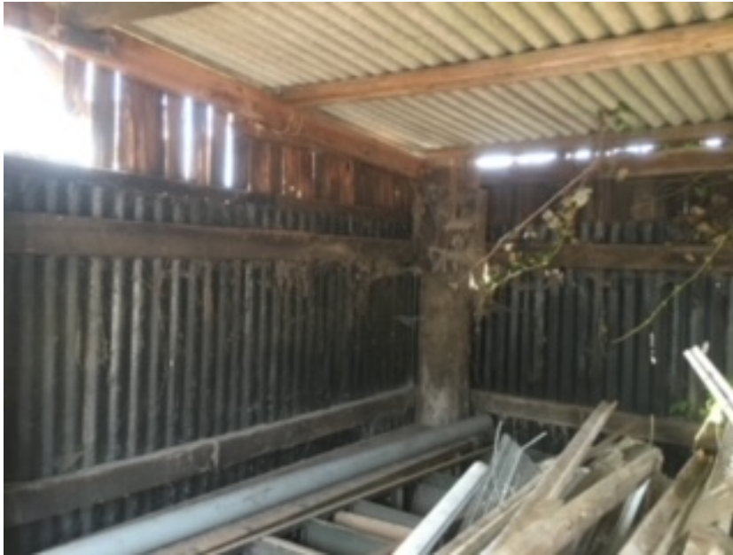
Corrugated walls on rear of cart hovel on solid supporting posts
