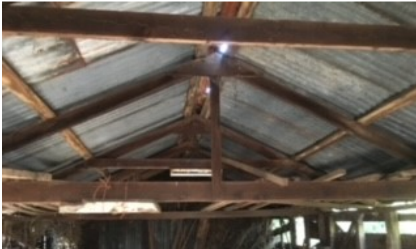
Timber trussed roof in tractor shed
