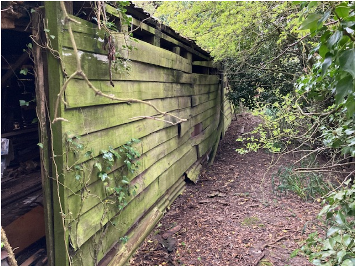
Cladded wall along front elevation
