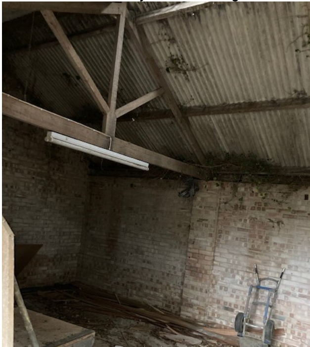
King post roof structure in stables/stores
