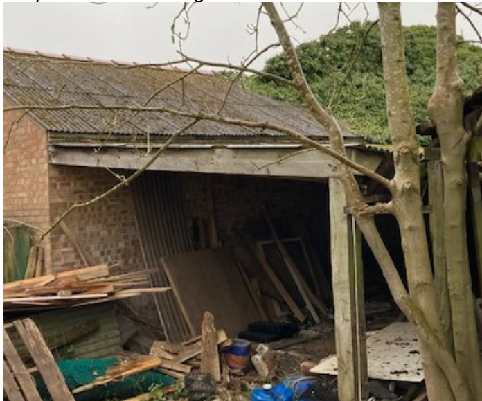
Supporting posts/rafters in implement store
