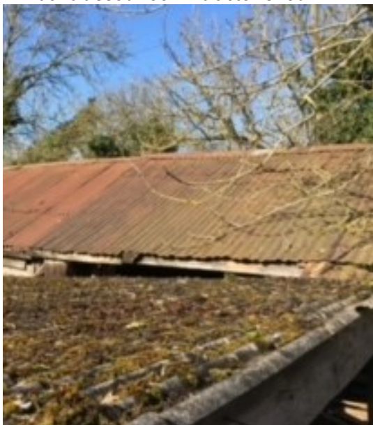
Corrugated roofs of outbuildings
