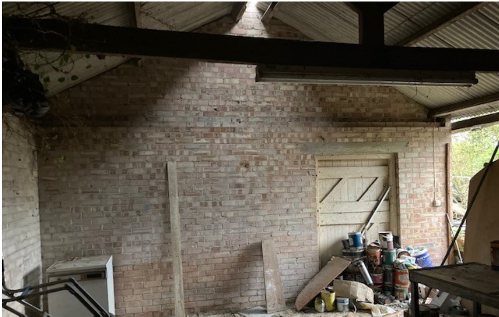
Stable door in masonry walls - looking onto workshop
