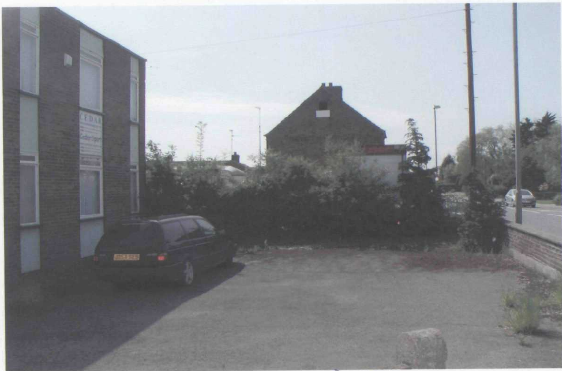
Site boundary with office & house to be demolished
