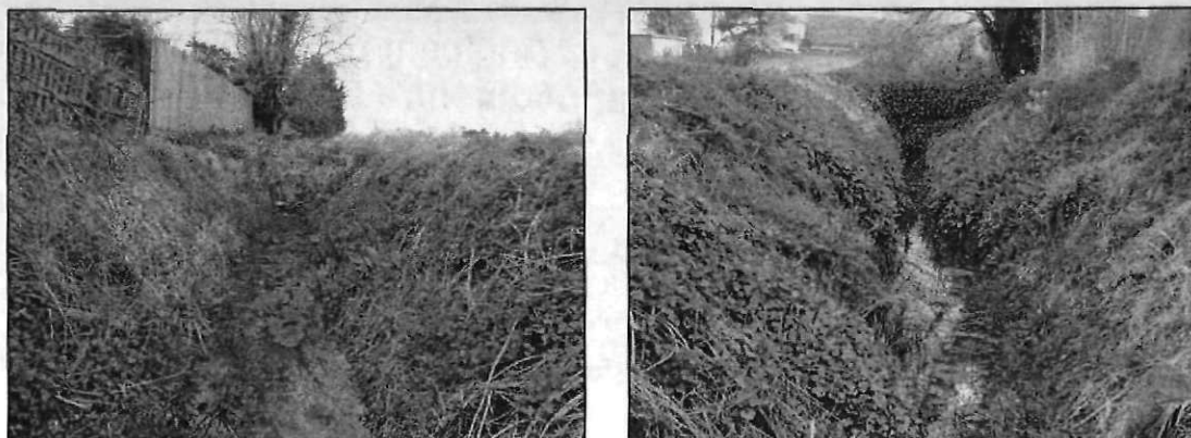
Photograph 1: Representative views of field drain showing the southern section looking north (left) and the northern section looking south (right).
