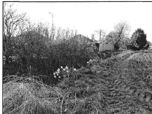
Photograph 5: [2] - Representative view of southern section of field drain looking north.
