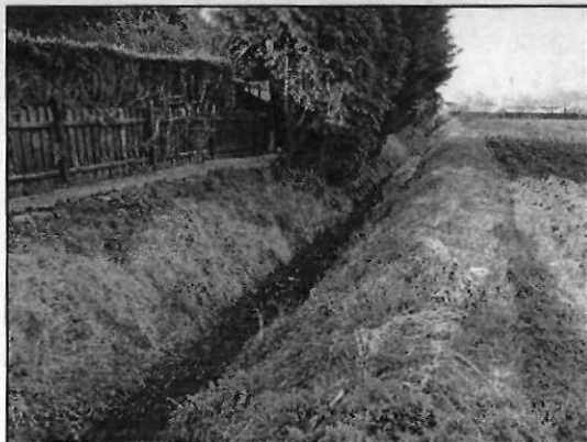
Photograph 10: [7] - Representative view of northern section showing wooden fencing and Leylandii boundary.
