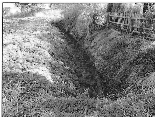
Photograph 7: [4] - Representative view of the southern section looking south from infill section.
