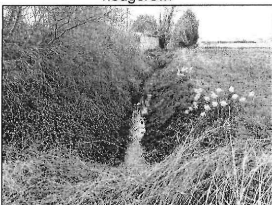
Photograph 6: [3] - Representative view of the southern field drain looking north,
