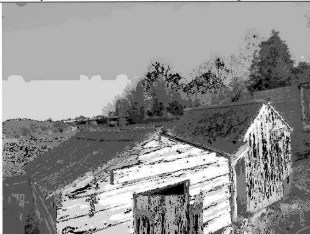
12. Partially collapsing shed adjacent to tanks X 2 with ACM roofing
