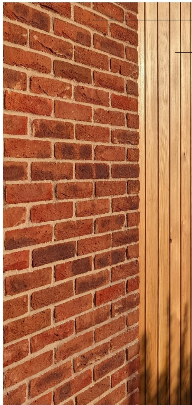
Red facing brickwork
