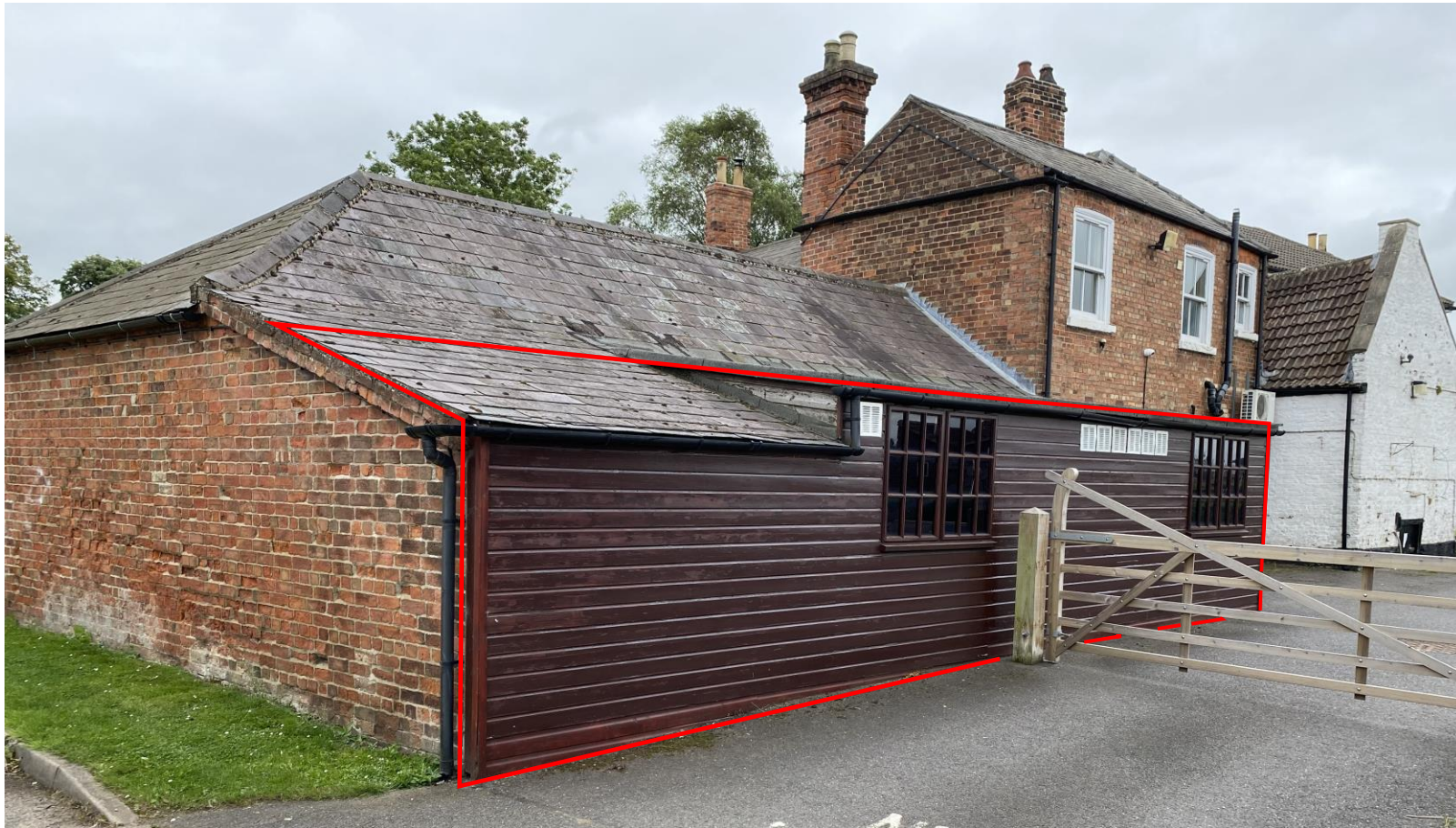
Kitchen Lean-to (area to be demolished) adjacent Stockhouse Lane entrance
