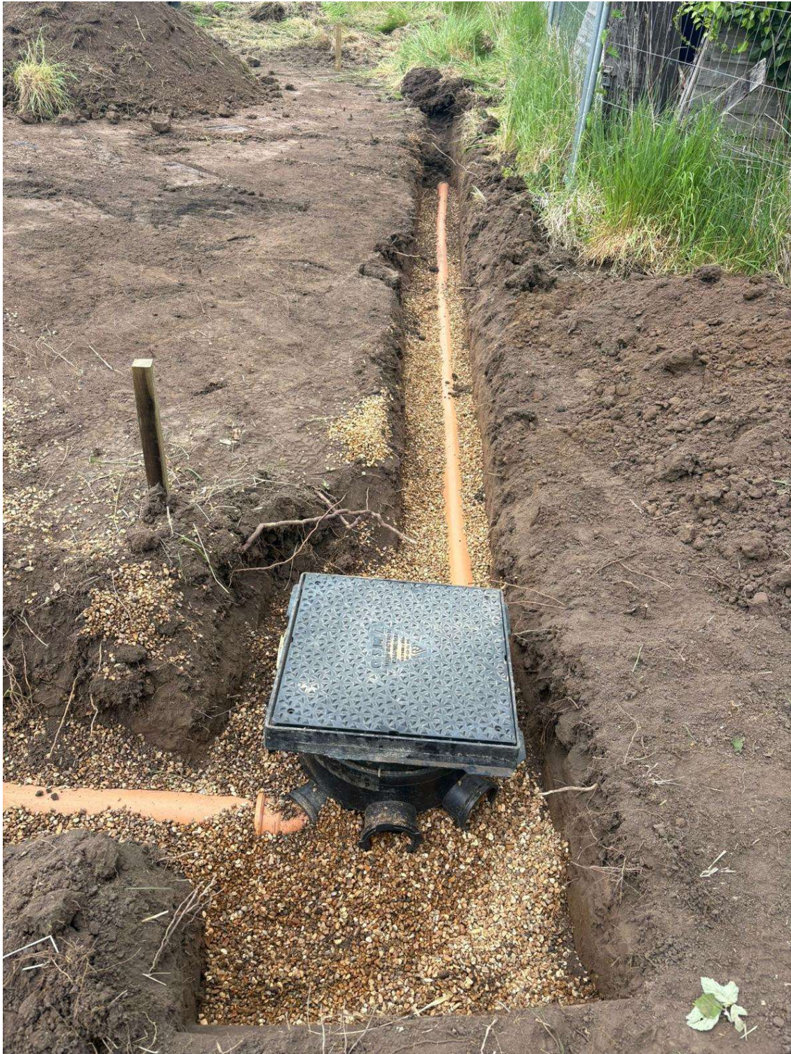
Photograph of new manhole installed.
