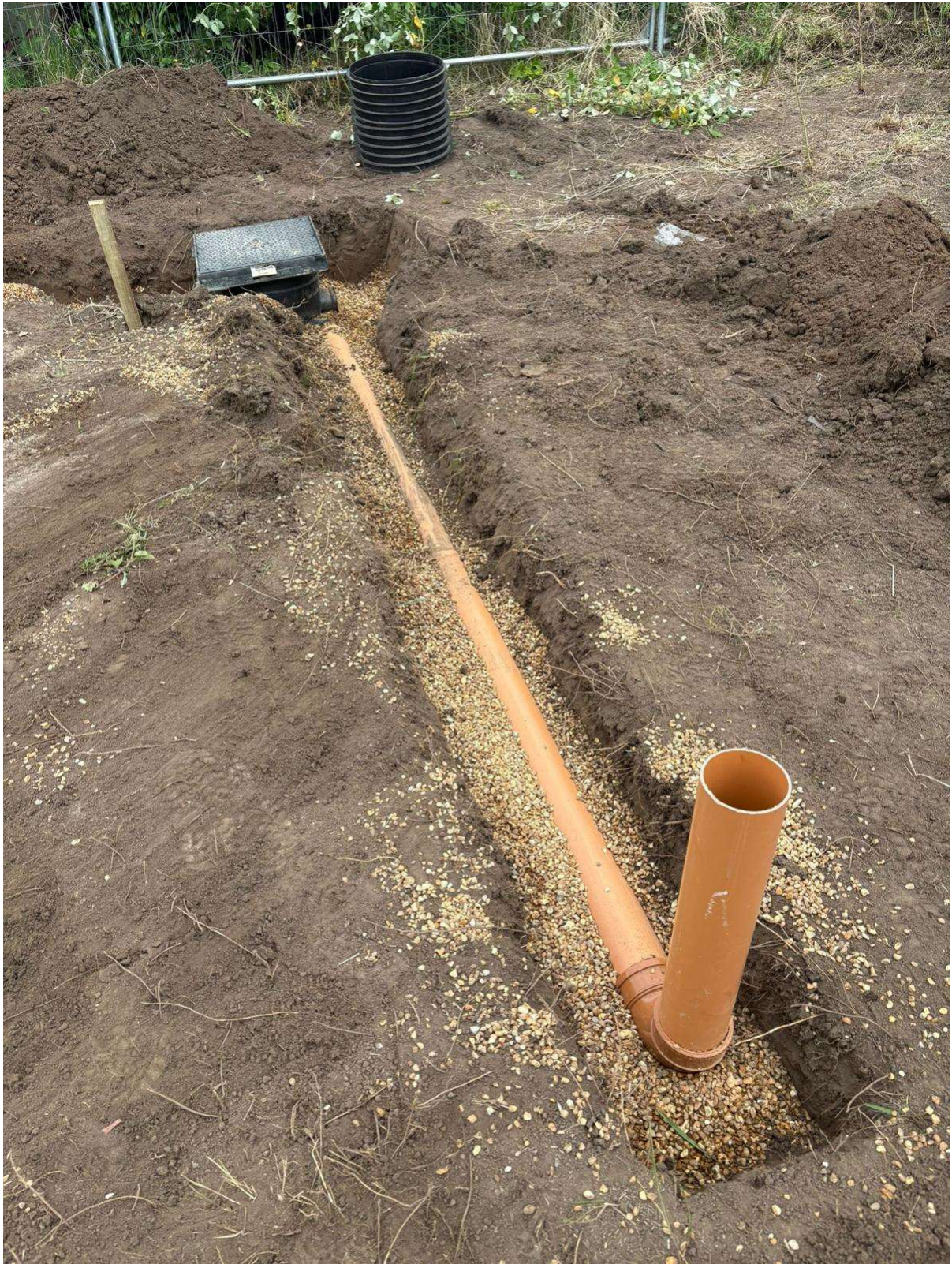
Photograph of new waste pipe installed.
