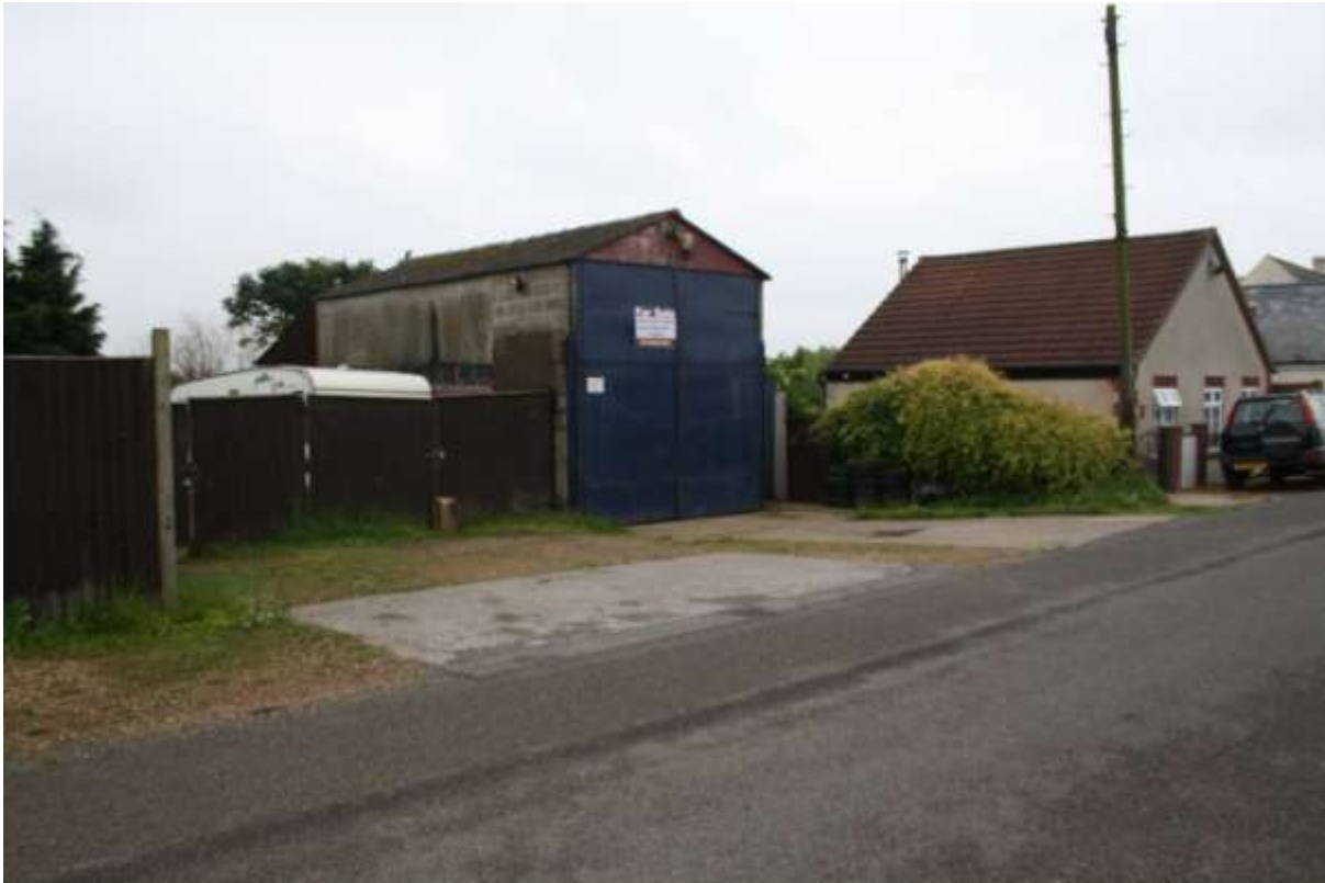
Proposed site from Reservoir Road
