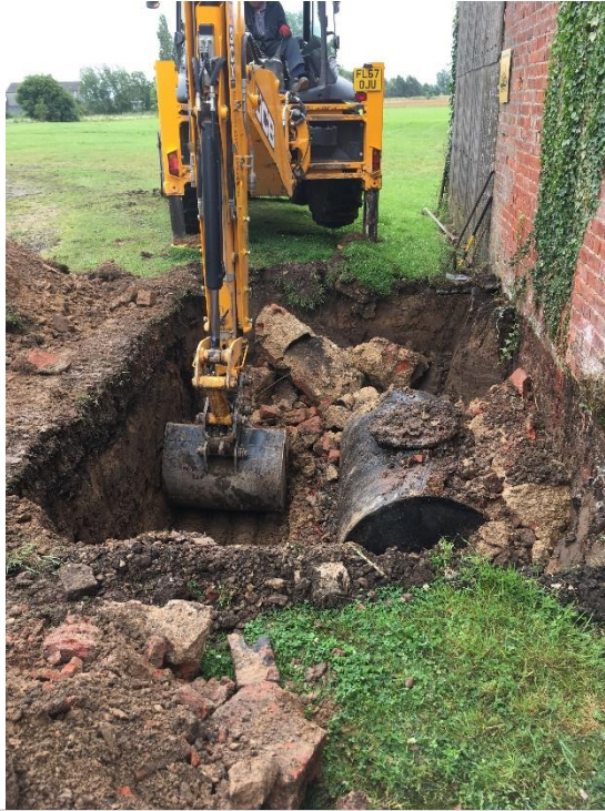
Underground storage tank exposed
