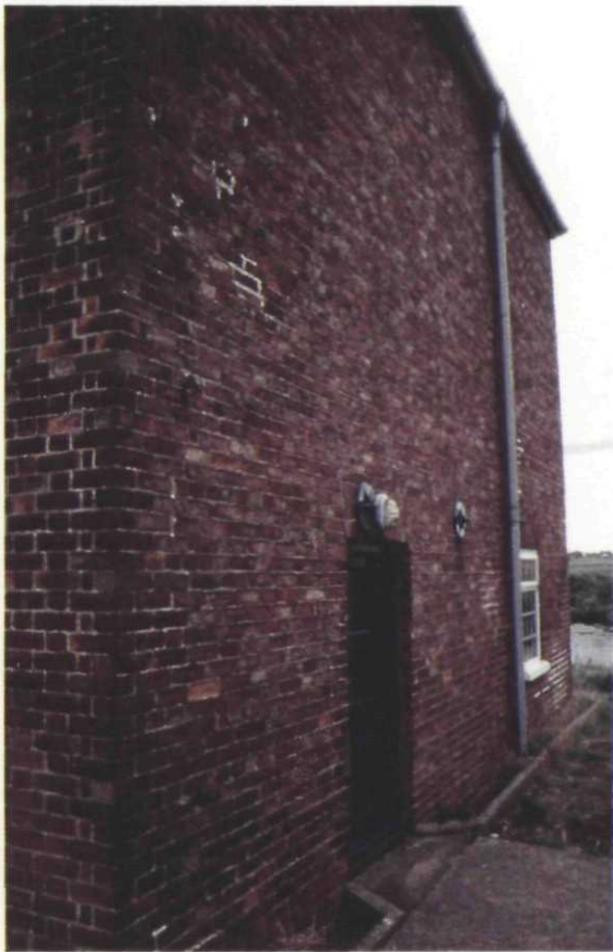
Plate 4 West elevation, looking south
