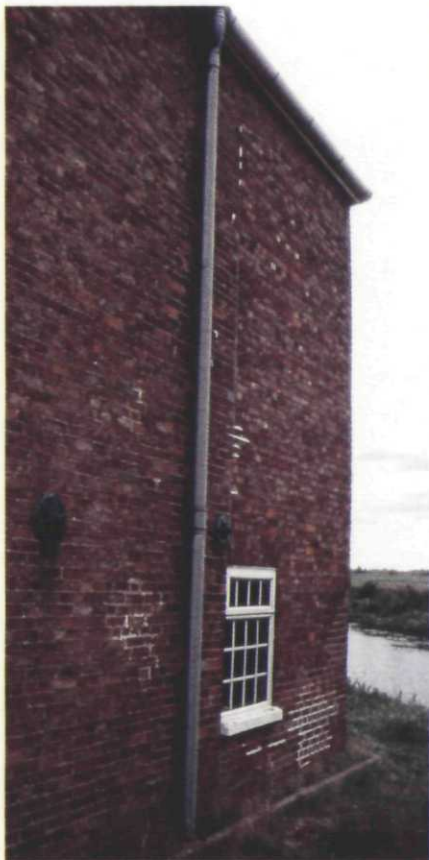
Plate 6 West elevation, showing straight join
