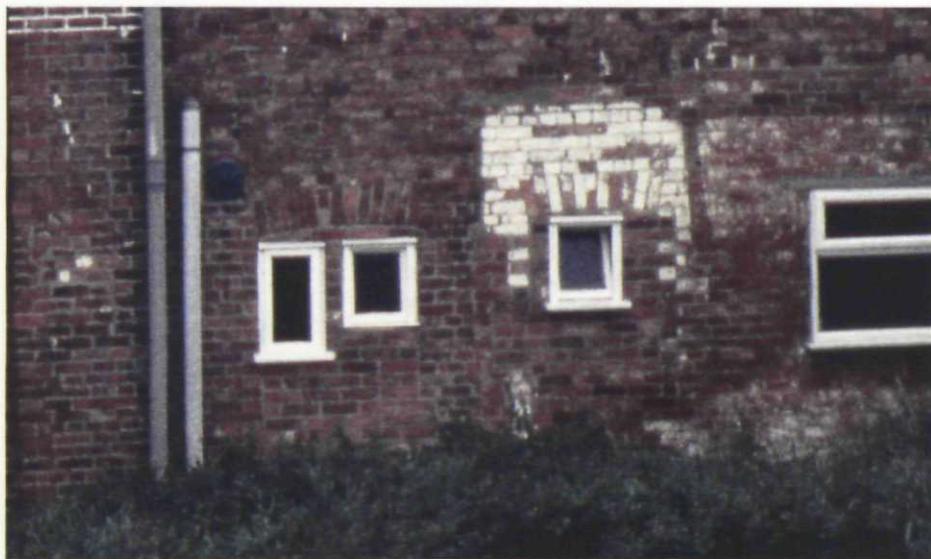
Plate 8 South elevation, showing blocked door and window
