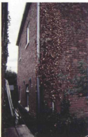
Plate 9 East elevation, looking south
