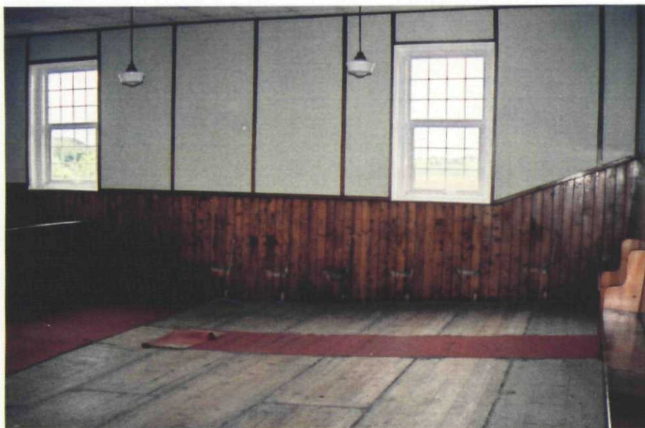
Plate 13 Church, panelling, showing scars of removed pews
