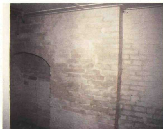
Plate 21 Alcove in utility area
