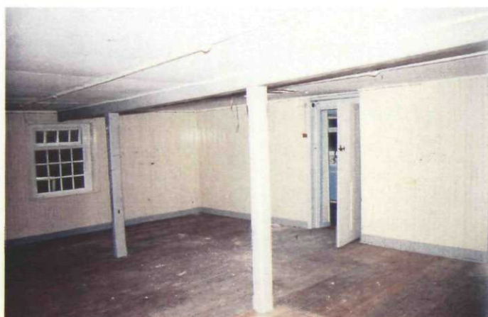
Plate 20 Lower level meeting room, showing stanchions, beam and door to utility area
