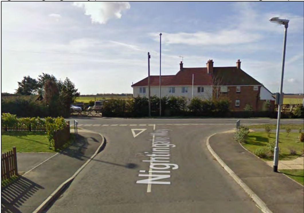
Figure 3: Nightingale Way (View Southbound Towards Junction with Bridge Road)
