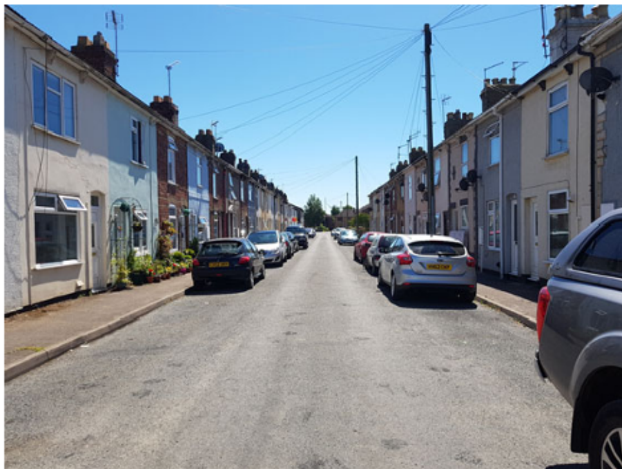
View Looking South along Withington Street.
