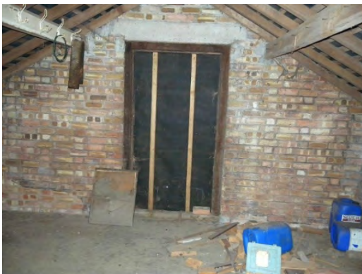
Photograph 4: Interior of upper storey, blocked up door on eastern elevation
