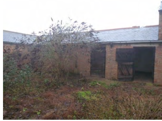
Photograph 11: Southern elevation of northern stores
