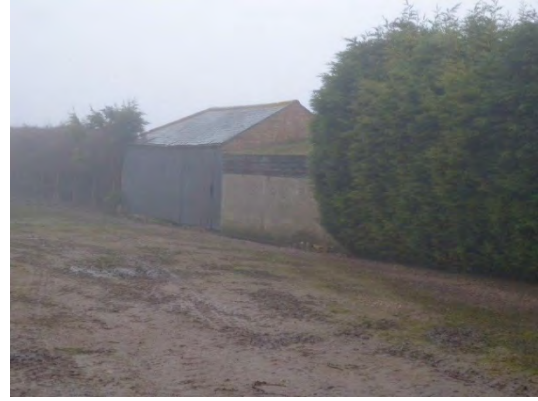
Photograph 13: Western elevation of cart-sheds
