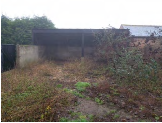
Photograph 12: Eastern elevation of southern cart-shed, concrete wall at south of site enclosing courtyard area
