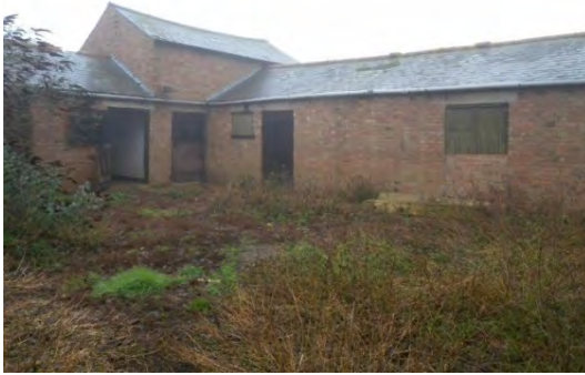
Photograph 6: View of two-storey barn and eastern single storey barn from courtyard
