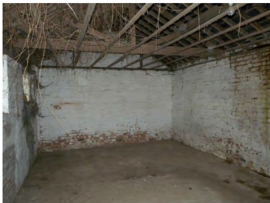
Photograph 8: Interior view of northern large store
