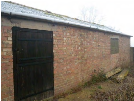
Photograph 2: Western elevation of eastern single storey barn
