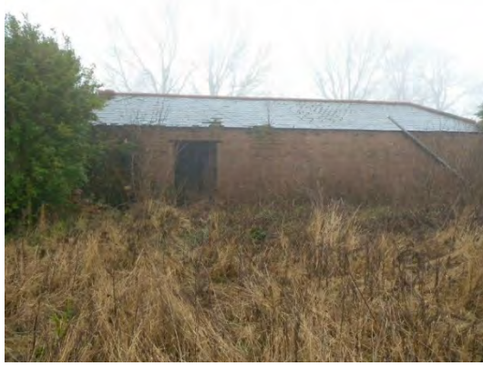
Photograph 10: Northern elevation of northern stores
