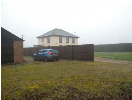
Photograph 19: Adjacent house with slate covered roof
