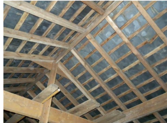
Photograph 3: View of roofing on eastern single storey barn
