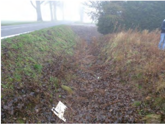
Photograph 17: Dry ditch on southern boundary
