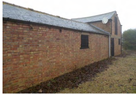
Photograph 7: Eastern elevations of eastern single storey barn and two-storey barn
