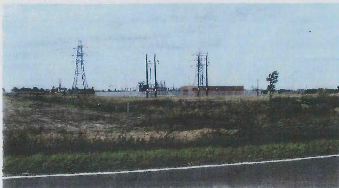
Power distribution infrastructure south of Holbeach
