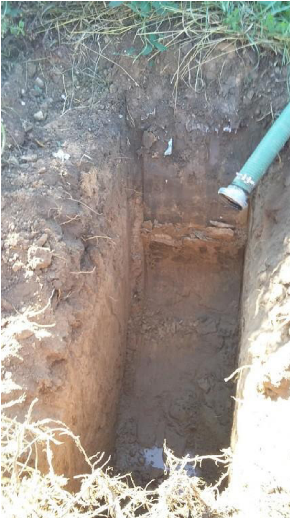
Photograph 5: Trial pit TP2, immediately prior to filling.
