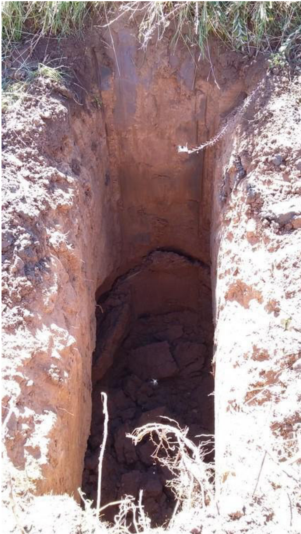
Photograph 6: Trial pit TP3, showing collapsing of saturated soil.
