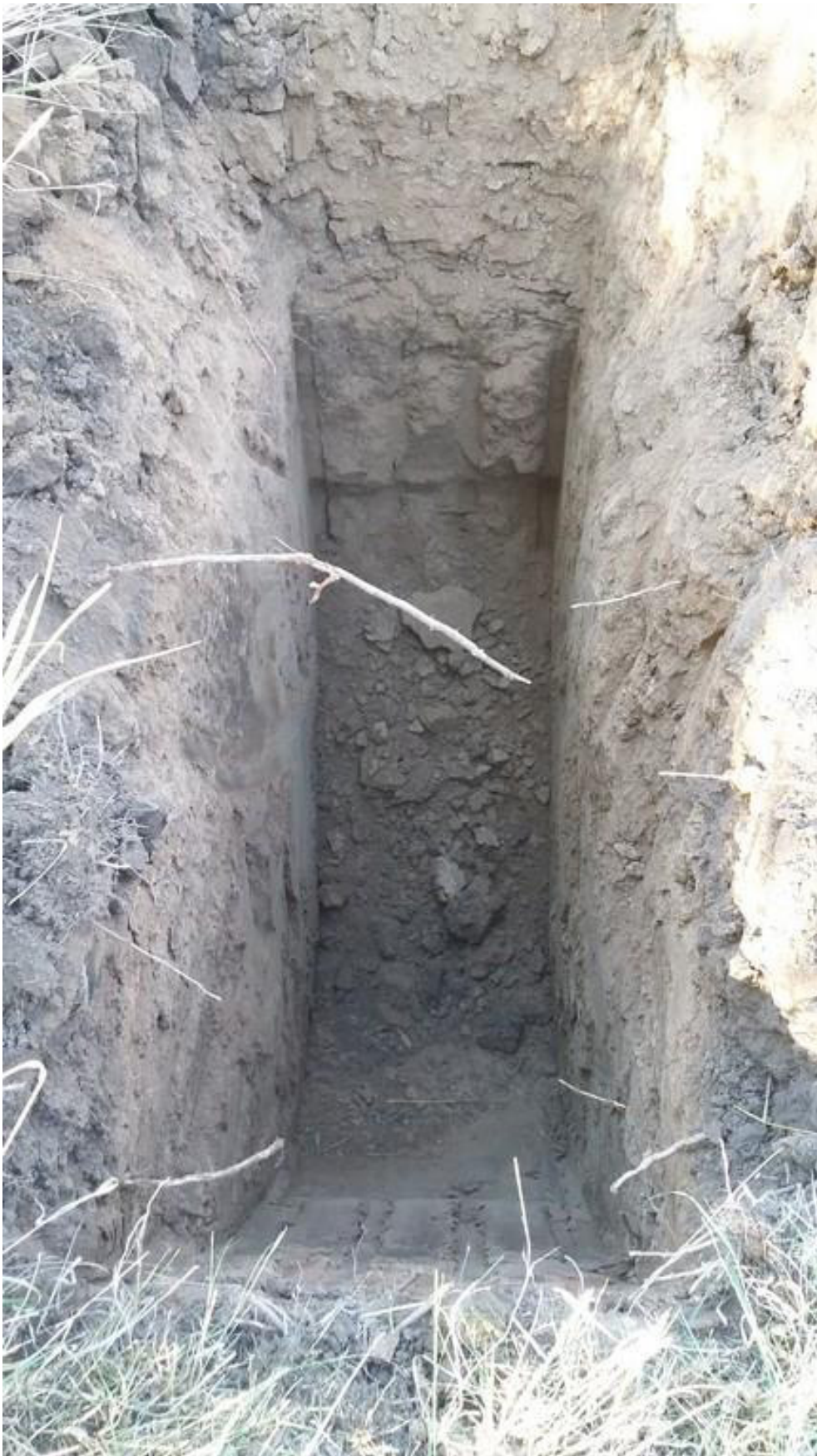
Photograph 11: Trial pit TP8
