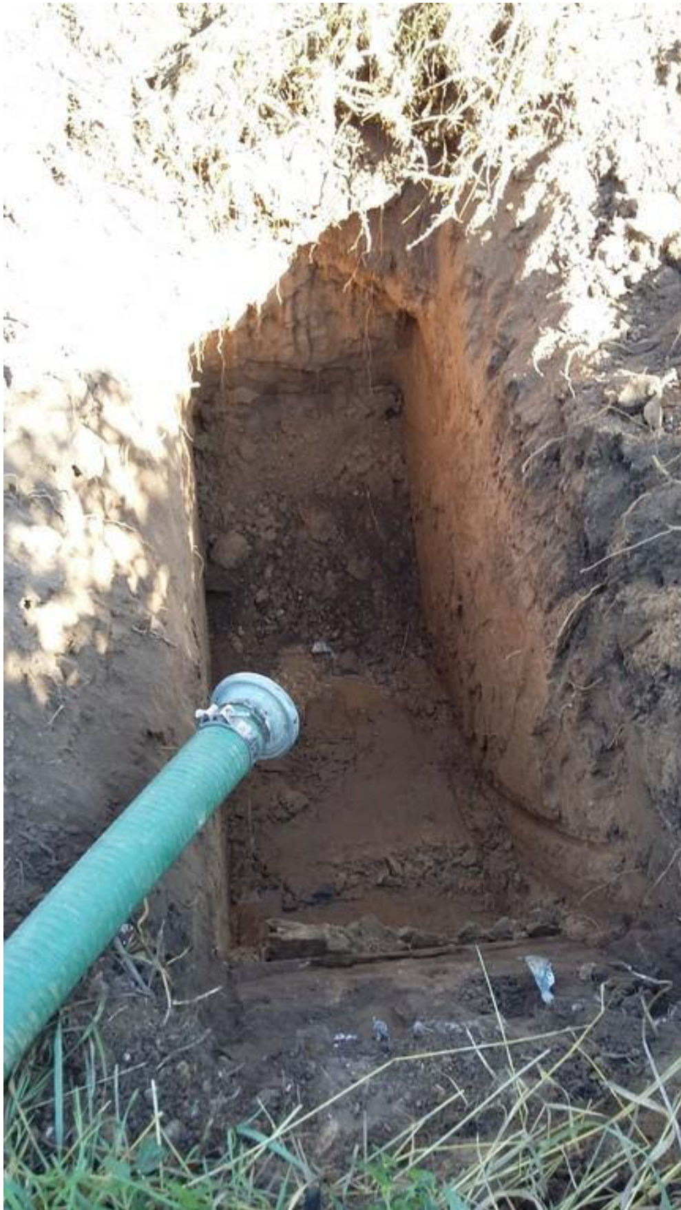
Photograph 4: Trial pit TP1 immediately prior to filling.
