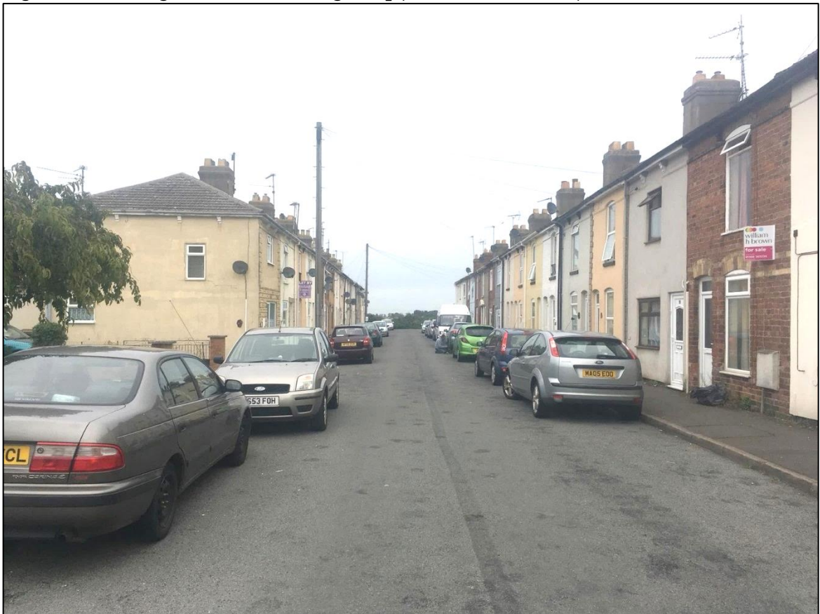
Figure 2: Withington Street Carriageway (view: northbound)
