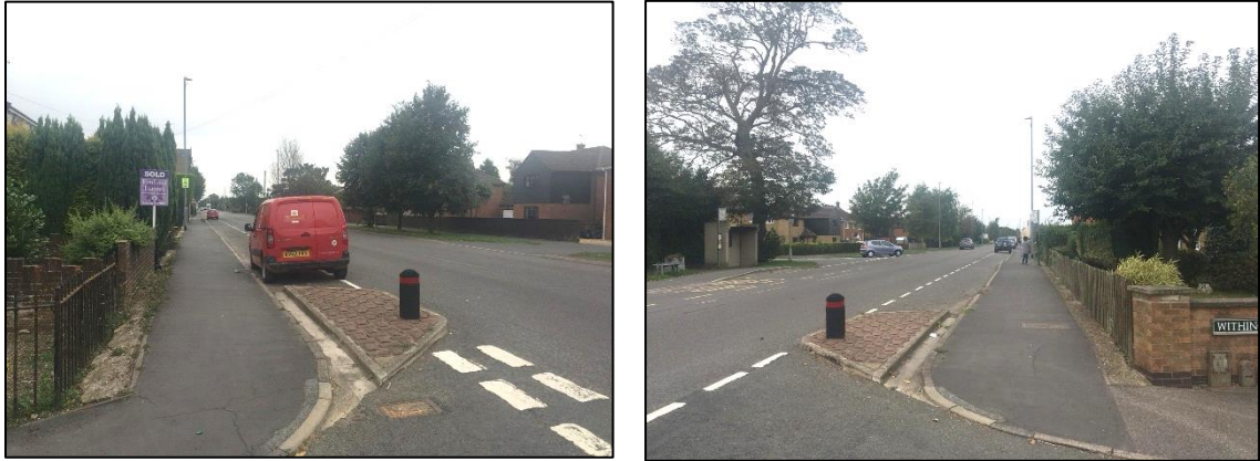
Figures 4 and 5: Withington Street/Bridge Street view
