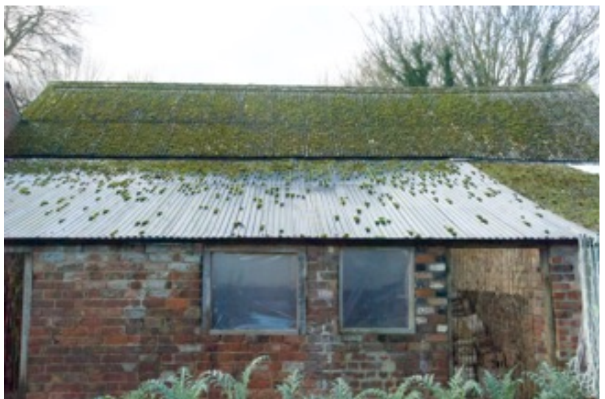
Plate 9 - View of Rear Elevation (B)
