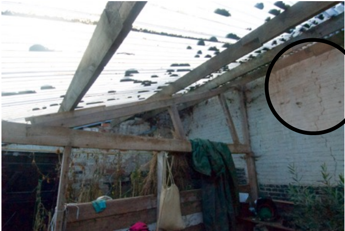
Plate 10 - Very simple timber rafters to support temporary roof.
