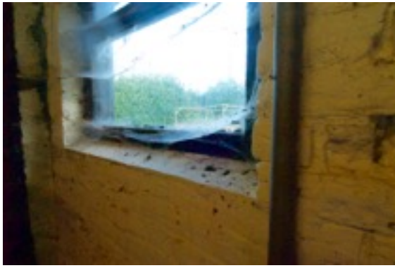
Plate 16 - Window detail showing historic changes
