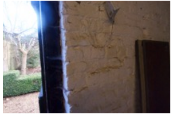
Plate 17 - Walls showing whitewashing for protection from decay.
