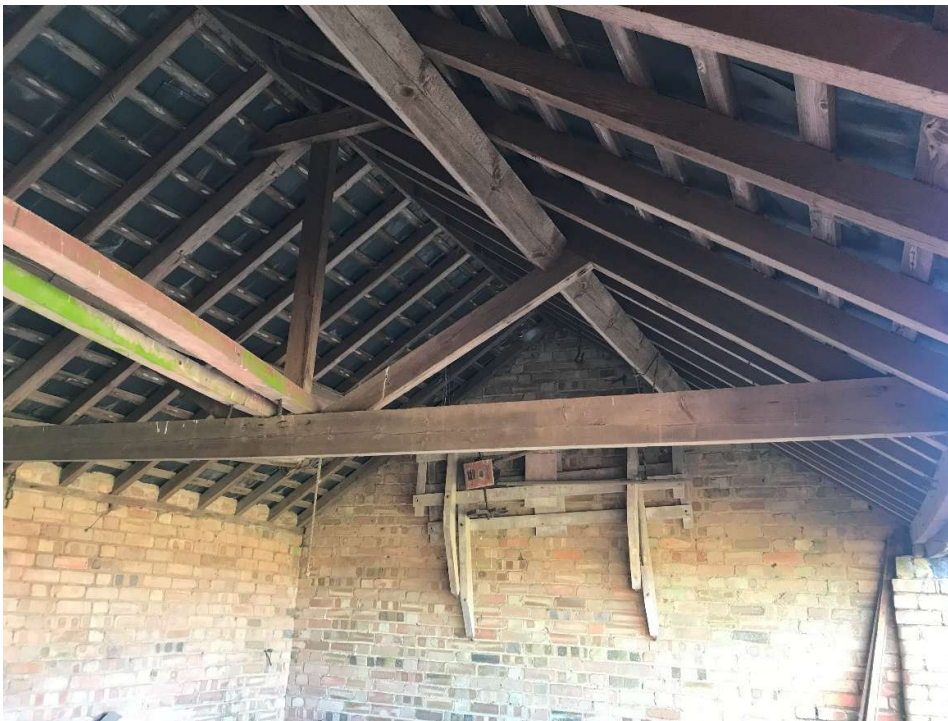
Photo 17. Store 4 king post roof truss
