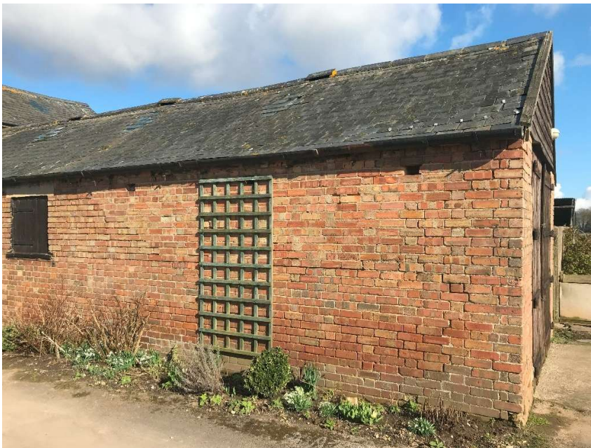
Photo 2. Store 1 west wide elevation – southern end
