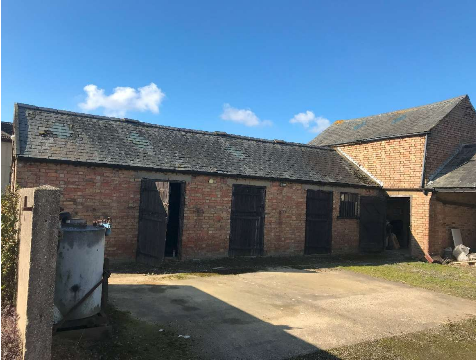
Photo 9. Courtyard Stores 1 and 2 side elevations
