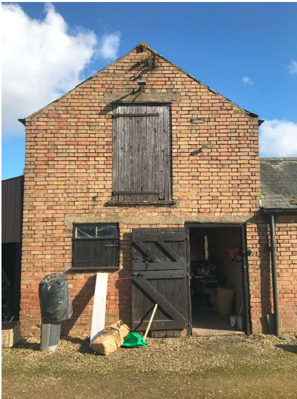
Photo 4. Store 2 west gable elevation
