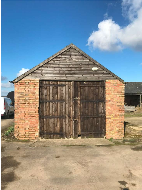
Photo 1. Store 1 front south gable elevation
