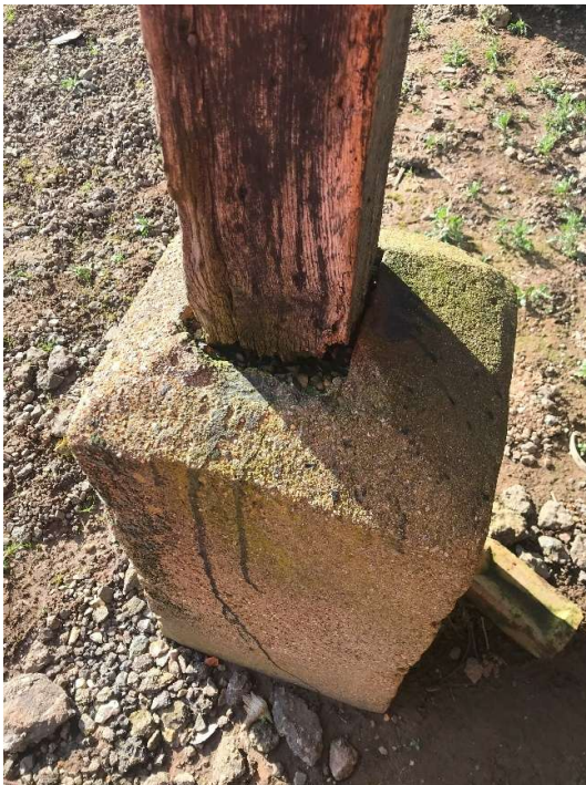
Photo 19. Store 3 timber post base detail
