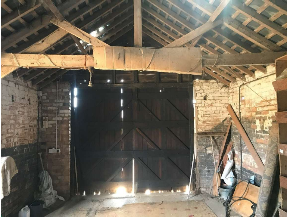
Photo 14. Store 1 king post roof truss
