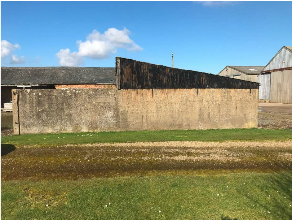
Photo 8. Store 5 south side elevation
