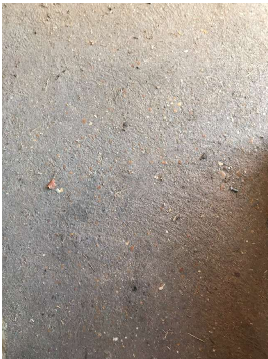
Photo 25. Store 2 concrete floor slab
