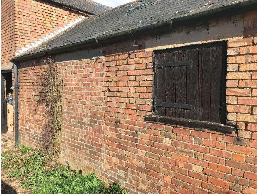
Photo 3. Store 2 west side elevation – northern end
