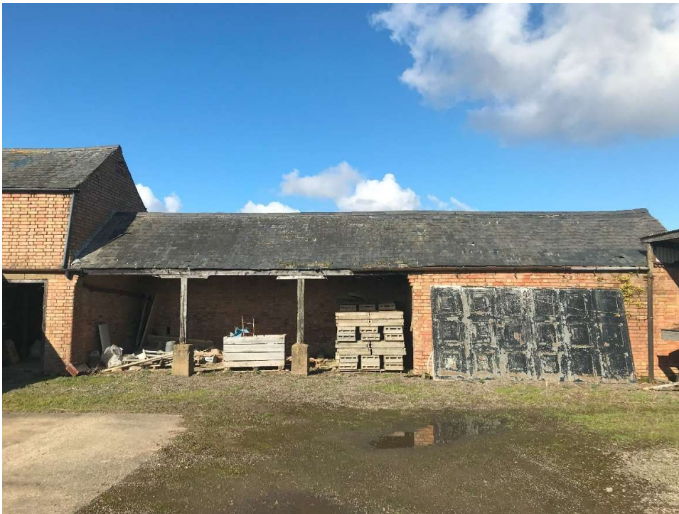
Photo 10. Courtyard Stores 3 and 4 side elevations
