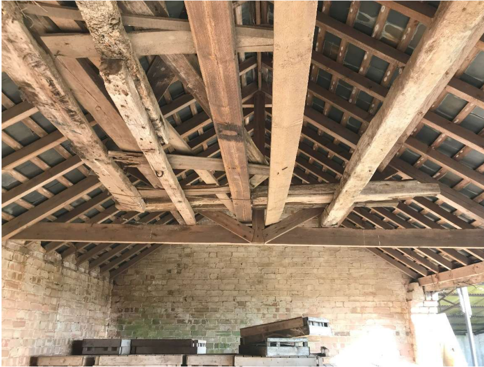
Photo 16. Store 3 king post roof truss
