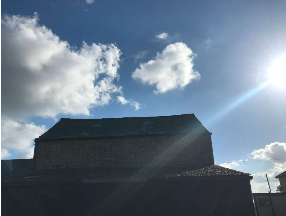
Photo 5. Store 6 north side elevation. Also Store 2 at first floor level.
