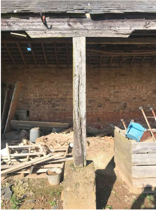
Photo 18. Store 3 timber post supporting eaves beam
