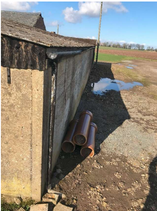
Photo 21. Store 5 east side elevation stormwater goods
