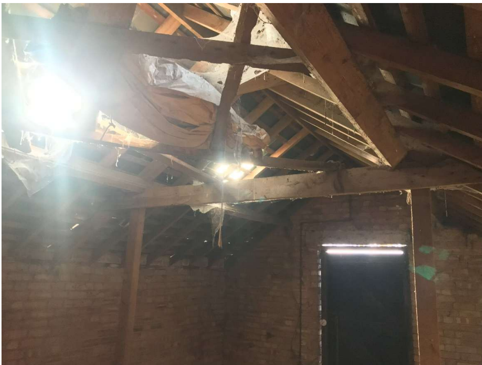
Photo 15. Store 2 king post roof truss
