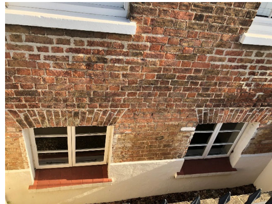
Dining Room windows looking down into light well from pavement to front of house
