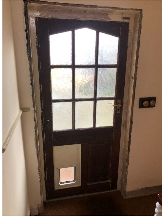
Rear entrance door (D1) – internal face
