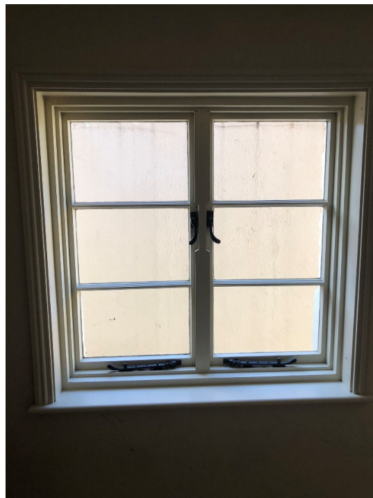
Dining Room window (W2) – internal face
