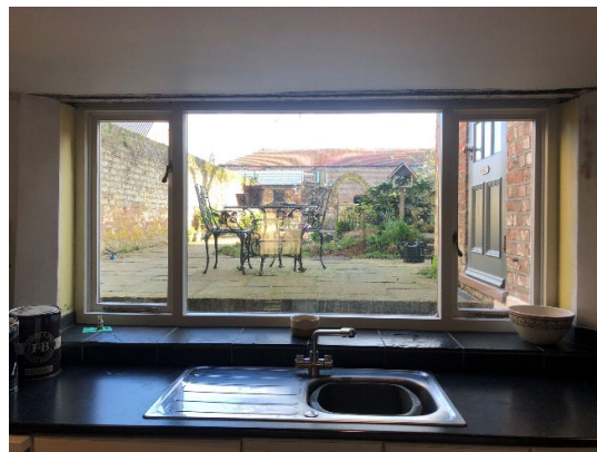
Kitchen window (W1) – internal face
