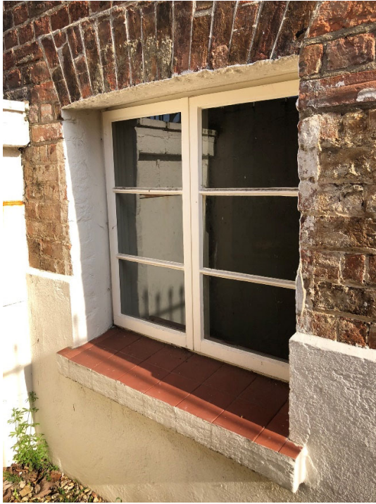
Dining Room window (W3) – external face
