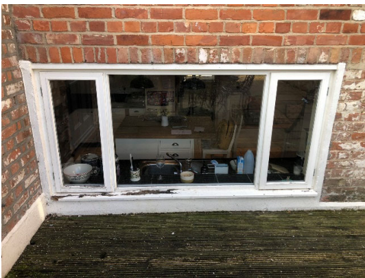
Kitchen window (W1) – external face
