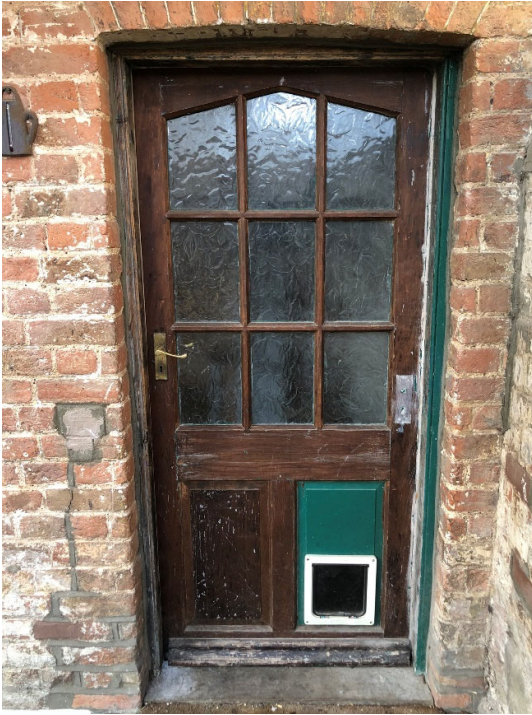
Rear entrance door (D1) – external face
