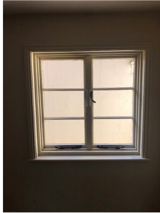
Dining Room window (W3) – internal face
