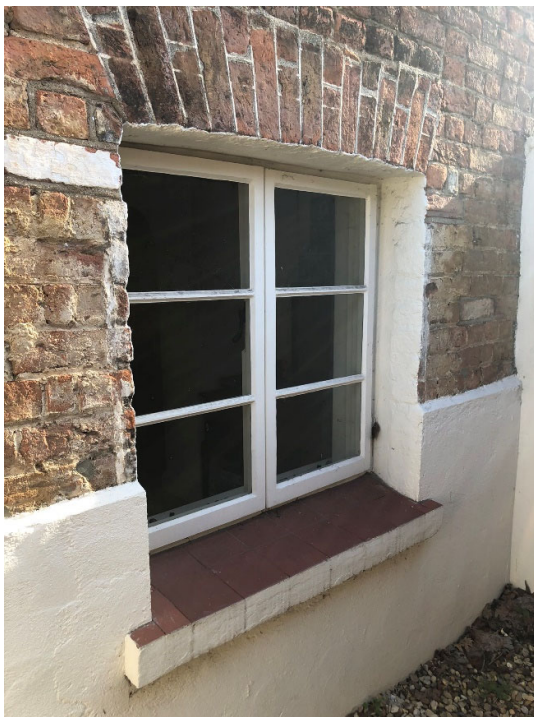
Dining Room window (W2) – external face
