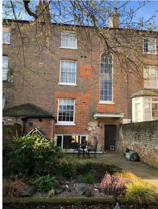
Rear elevation showing kitchen window and rear entrance door
