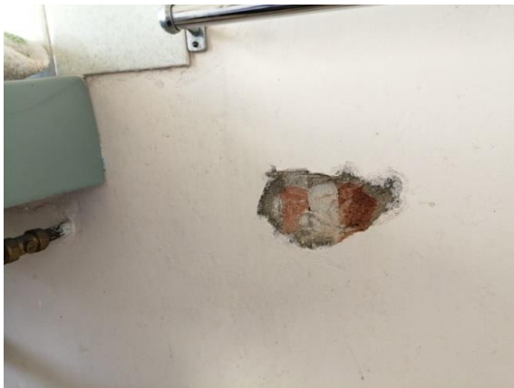
Sampling from toilet and bath dividing wall
