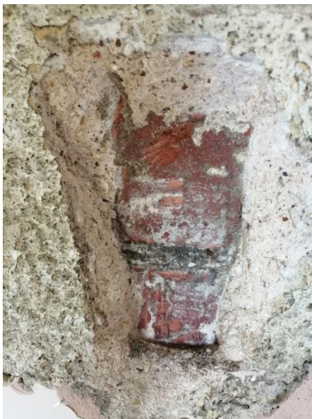
Sampling from shower cubicle wall.
