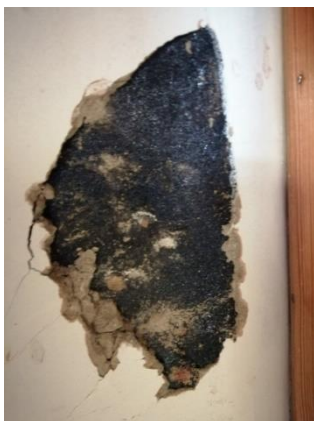
Clinker block, cement render, pink gypsum plaster skim
