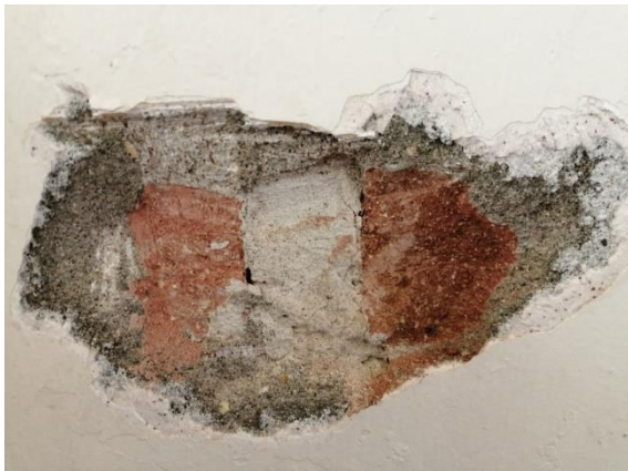
Pressed brick, cement render, pink gypsum plaster
