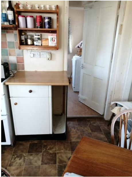
Kitchen partition wall
