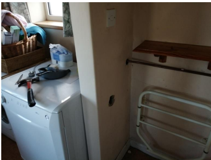
Corresponding wall with chiselled plaster
