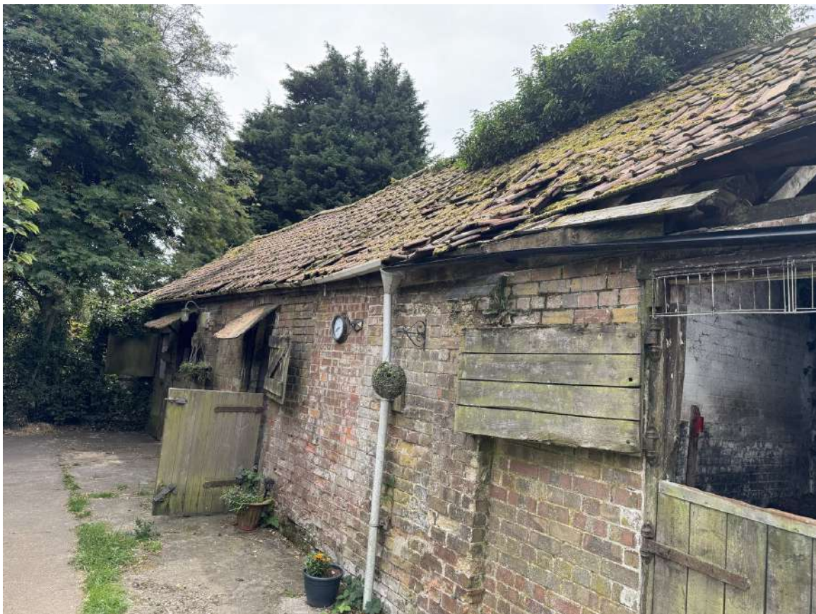
Image 1.0: Exterior view of barn complex showing open bay section with plain tile roof
