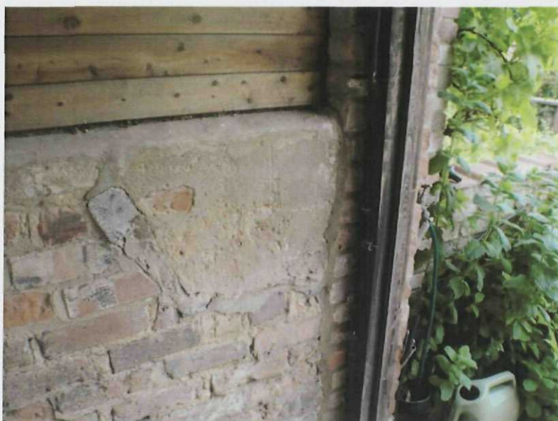
Plate 11. Visible in the west wall of Division C (in the entrance passageway to the courtyard) is the blocked remains of an integral manger within the wall. This suggests that Division C was for cattle accommodation
