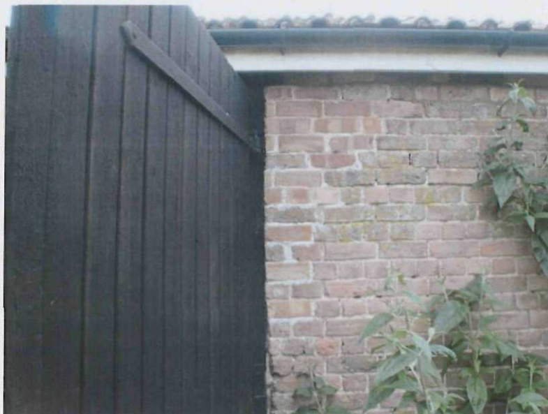
Plate 6. Detail of the brickwork on the eastern elevation of Division B. Note the ragged join by the door and the change from English to Stretcher bond in the upper portions of the wall.
