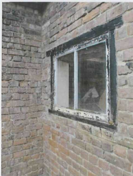
Plate 8 (above right). The north elevation of Division B, supported by a buttress. In both plates, the upper courses are laid in Stretcher bond where the roof height has been raised
