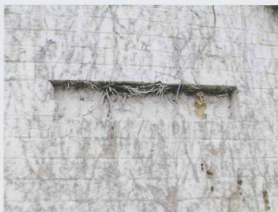
Plate 5 (Below). Detail of the recess in the brickwork on the eastern elevation
