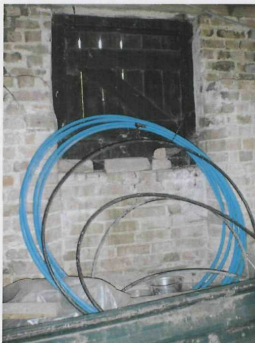
Plate 9 (Left). The raised window in the eastern elevation showing the chamfered aperture in the original wall. The alterations appear to have taken place when the roof was raised.
