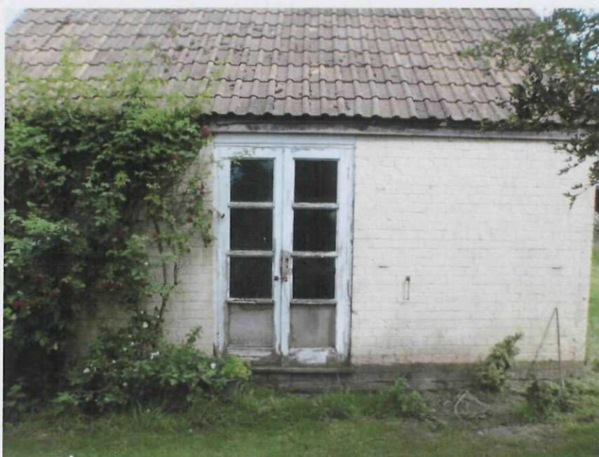
Plate 2. The southern elevation of Division A. This is one of the original walls of the latest addition to the structures comprising the southern range. It is constructed in English Garden Wall Bond.
