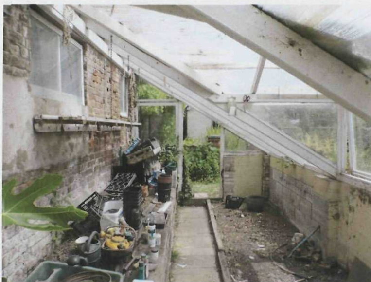
Plate 16. Internal view of Division, D, The Greenhouse. The breezeblock wall is attached to the main structure by angled timber joists forming a lean-to structure
