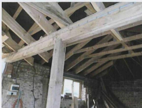
Plate 10 (Below). Various phases of roof timbers. The upper timbers are most recent and are attached to an older supporting timber and post
