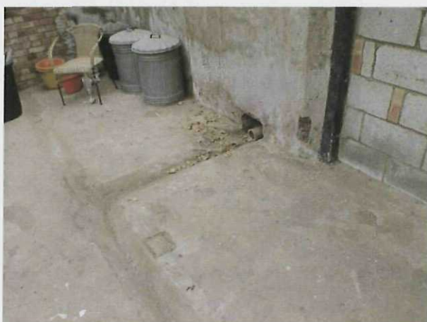
Plate 20. Detail of the manure drain with the outlet running into the central courtyard. It continues west, underneath the modern wall at the left of the picture
