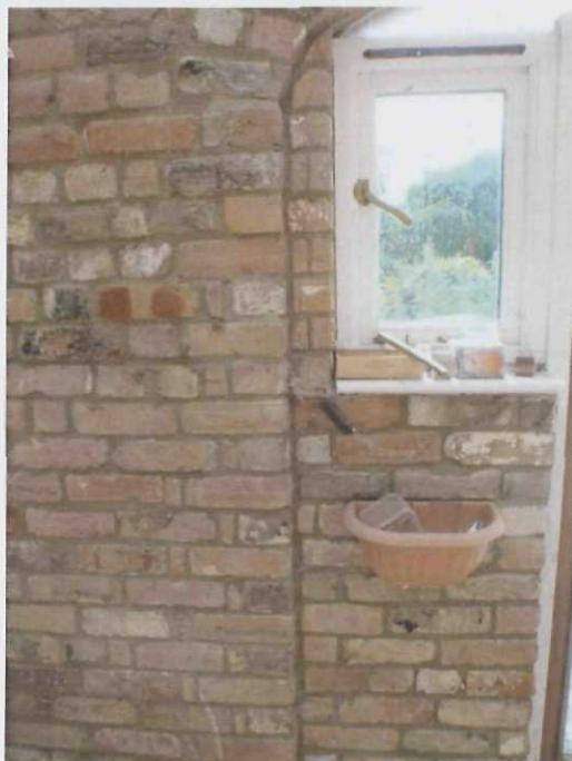
Plate 14 (Left). Internal detail of the decorative arched doorways, showing the new mortar and recent construction.
