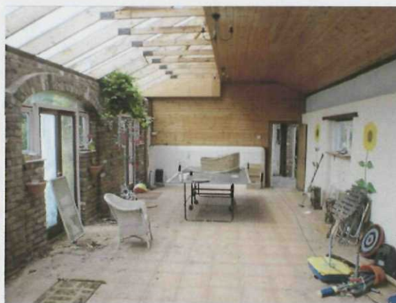
Plate 15 (below). Internal view of Division C showing the suspended ceiling and modern roof construction
