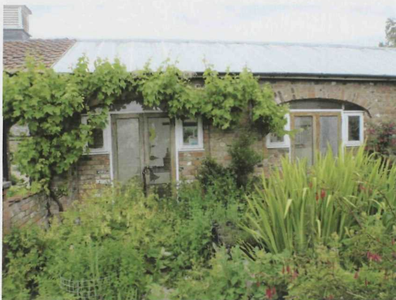
Plate 13. External view of the south elevation of Division C showing the decorative arched entranceways.
