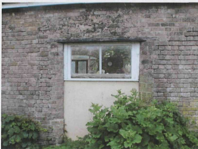
Plate 12. The blocked doorway in the northern elevation of Division C. The upper six courses, laid in stretcher bond show the alteration to the roof height. The brickwork around the chamfered door aperture shows evidence of repair or alteration
