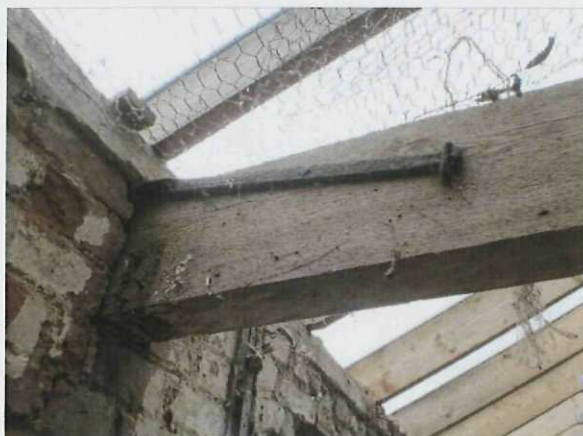
Plate 22. Detail of the roof timber and iron tie that appear to be contemporary with the original raising of the roof
