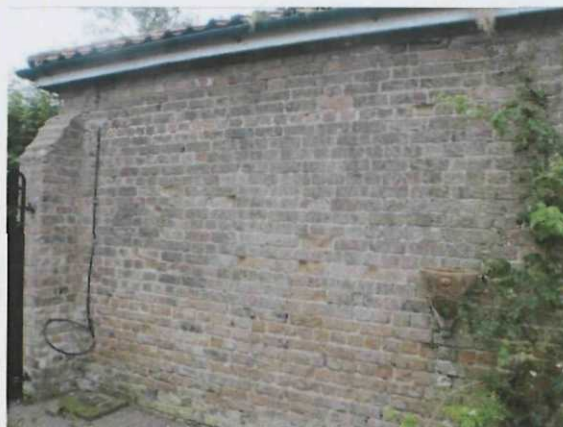
Plate 8 (above right). The north elevation of Division B, supported by a buttress. In both plates, the upper courses are laid in Stretcher bond where the roof height has been raised
