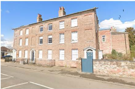
2. 64, 66 AND 68, BRIDGE ROAD
