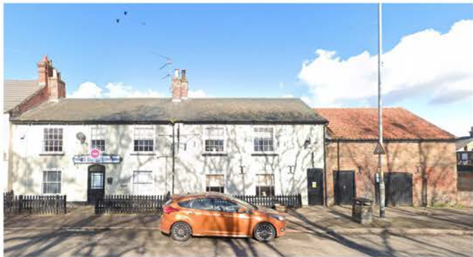
4. 8 AND 10, BRIDGE ROAD
