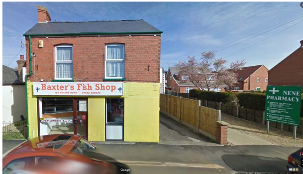
Front view of the site
