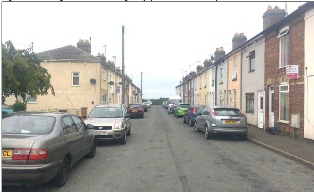
Figure 4: Withington Street Carriageway (View Northbound)
