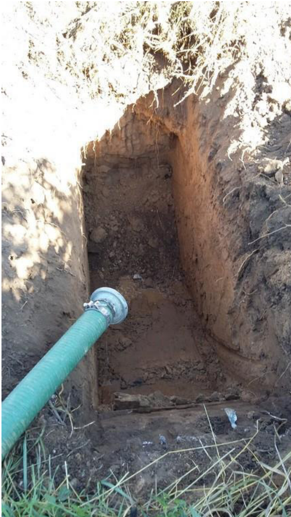
Photograph 4: Trial pit TP1 immediately prior to filling.
