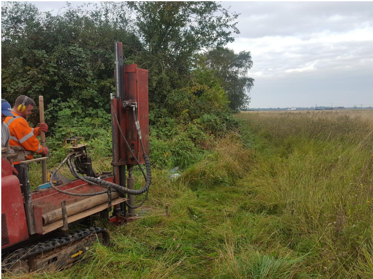
Photograph 2: Location of window sample hole WS5, facing north west. The white van is parked at the western end of Area C. The drill rig is positioned within Area B.
