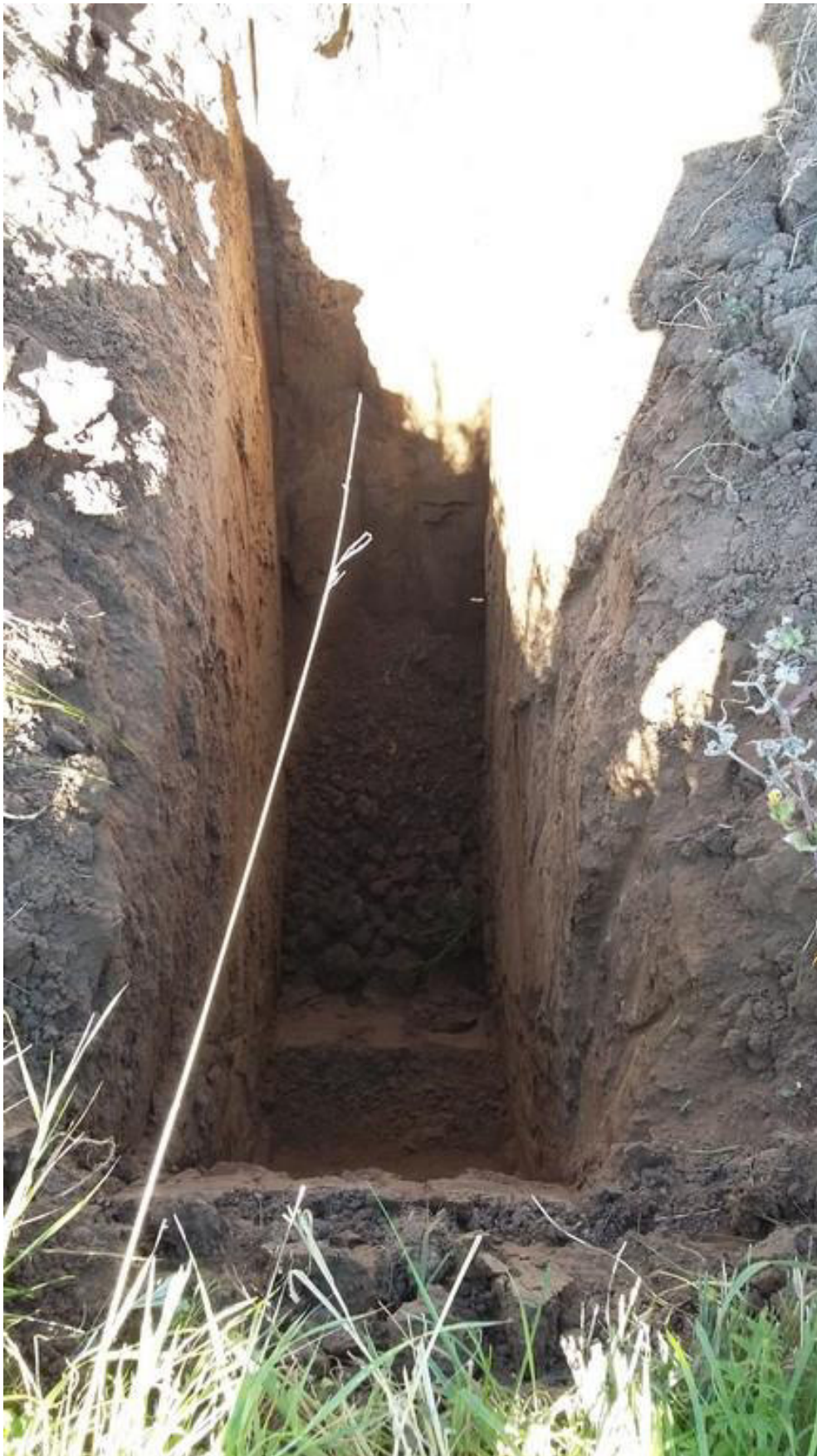
Photograph 8: Trial Pit TP5.
