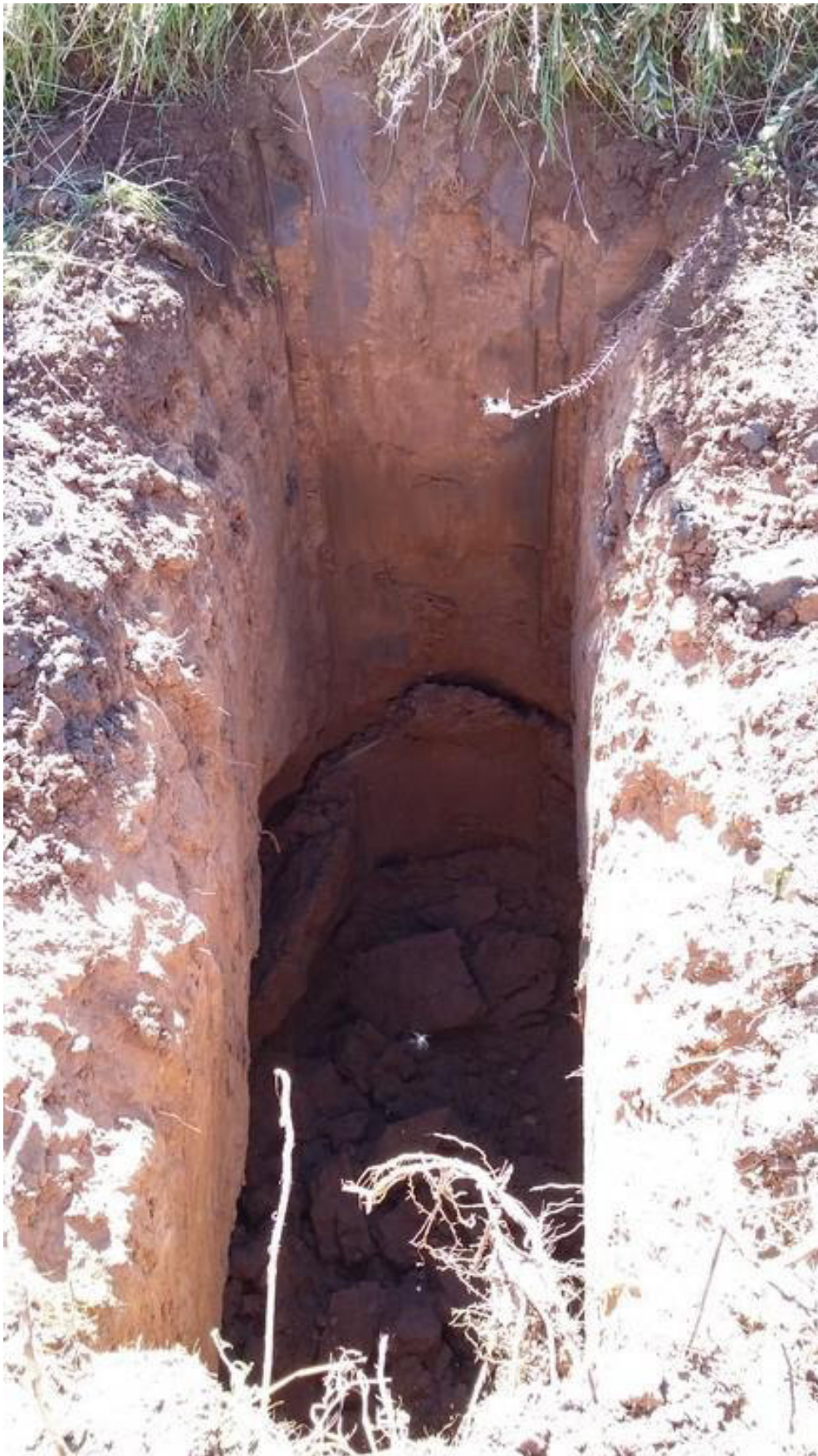
Photograph 6: Trial pit TP3, showing collapsing of saturated soil.
