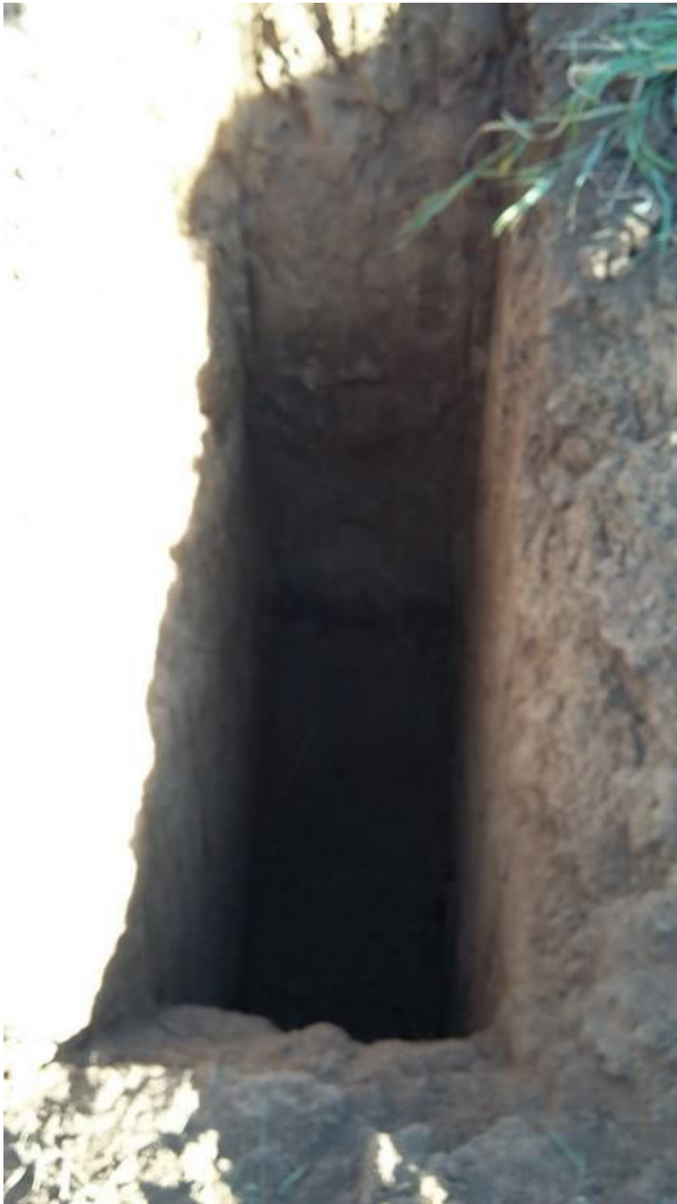
Photograph 10: Trial pit TP7
