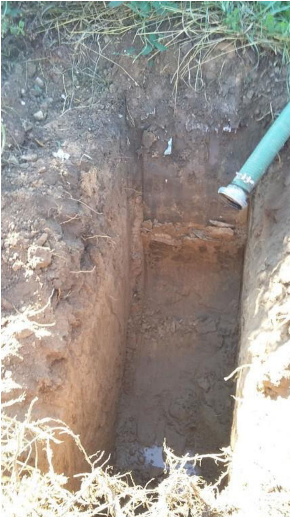
Photograph 5: Trial pit TP2, immediately prior to filling.
