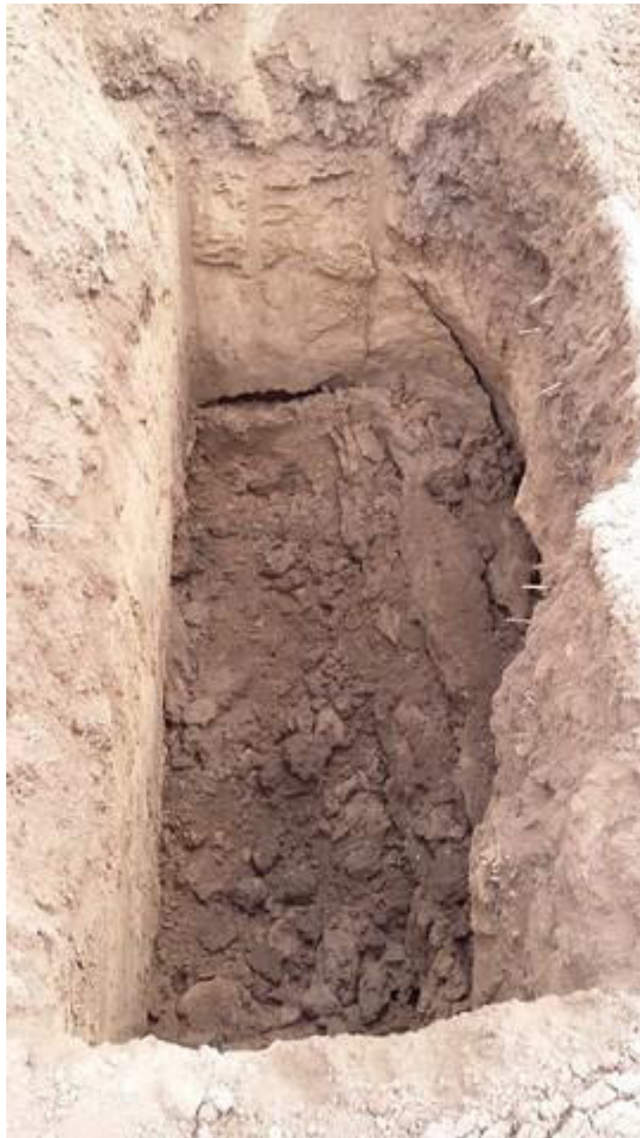
Photograph 10 – Trial Pit TP6
