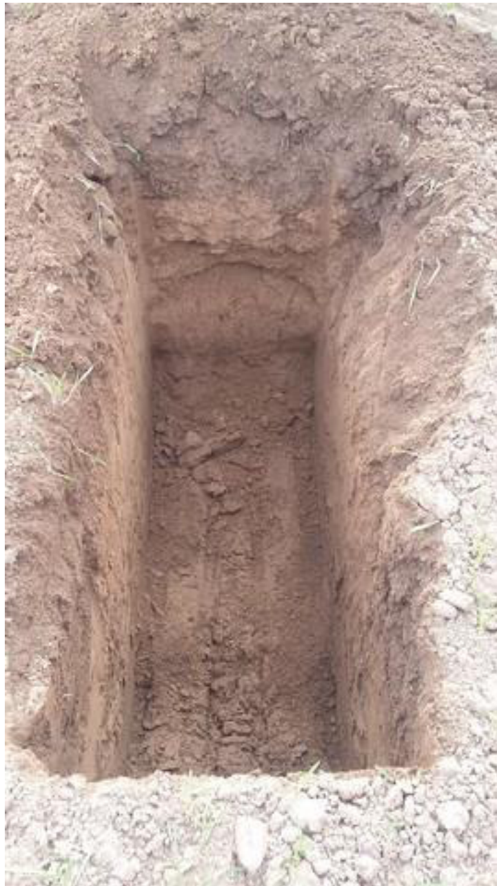
Photograph 7 – Trial Pit TP2
