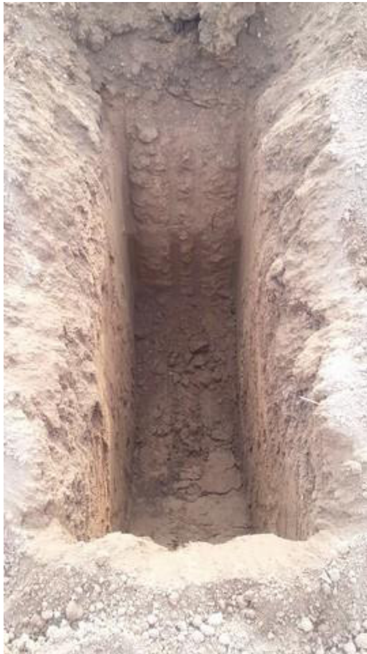
Photograph 6 – Trial Pit TP1
