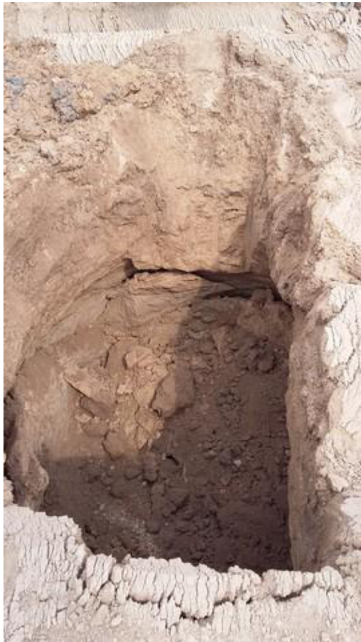
Photograph 8 – Trial Pit TP4
