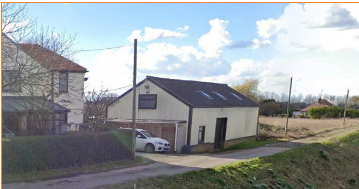
Figure 2: Site frontage (Source: Google Earth)
