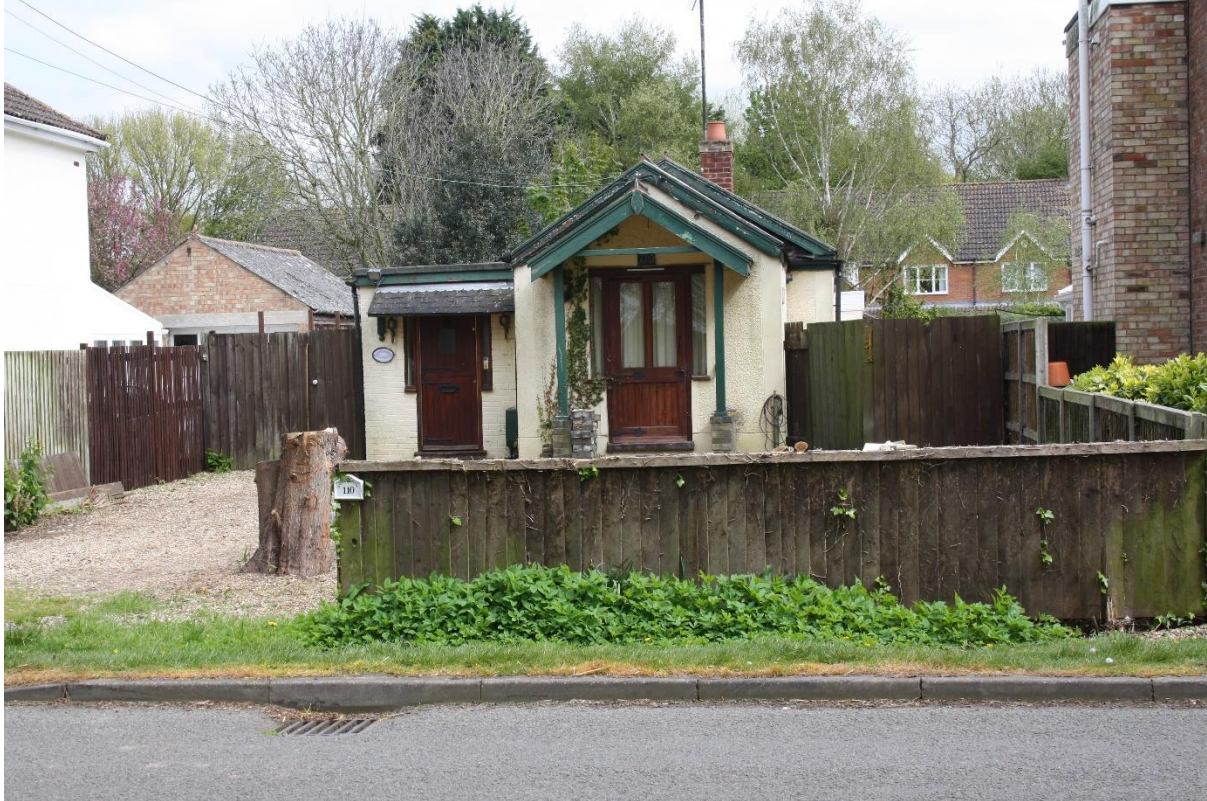
View of existing bungalow from New Road
