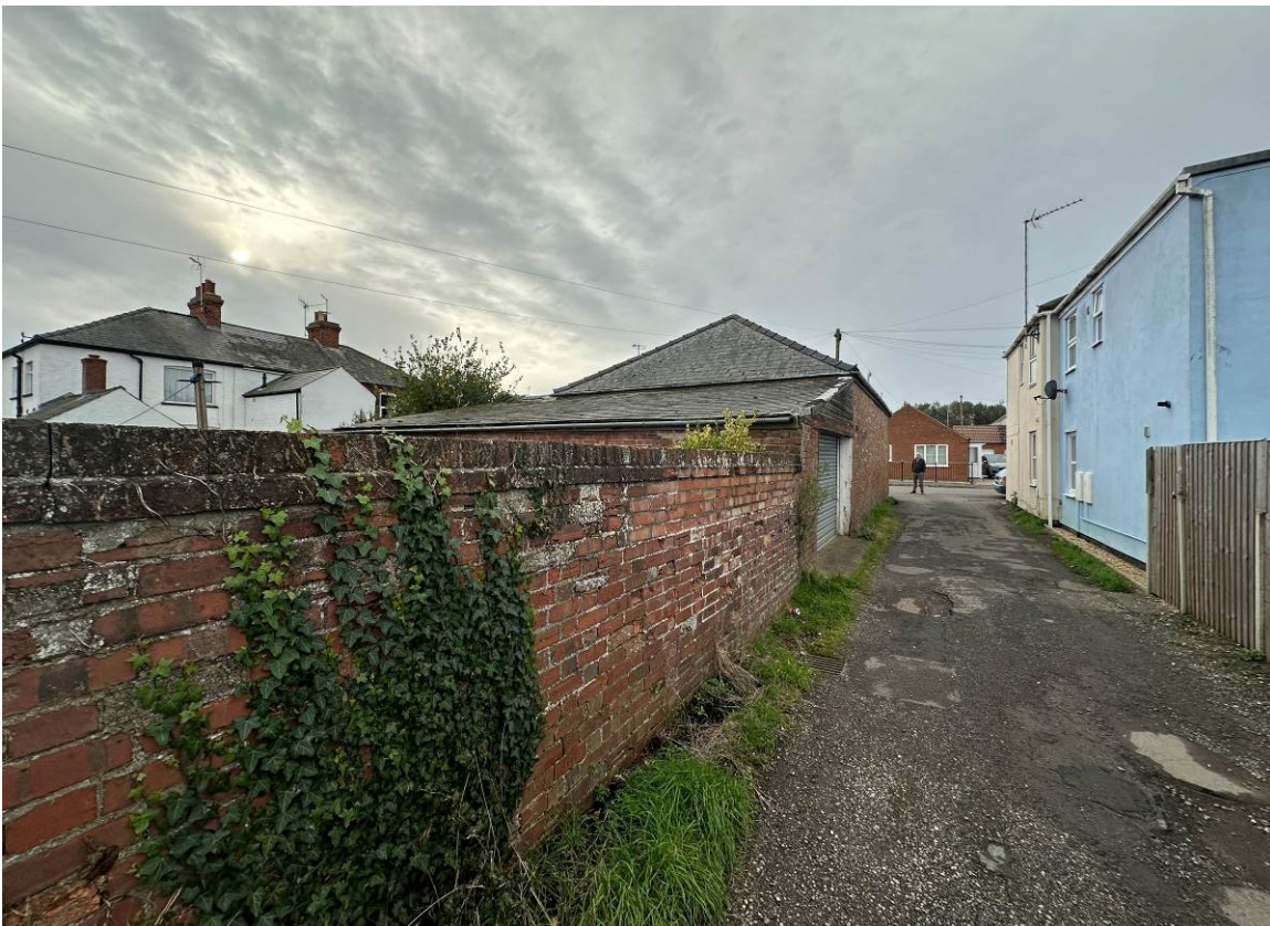
Rear/Side view of existing building from side street, looking towards King Street
