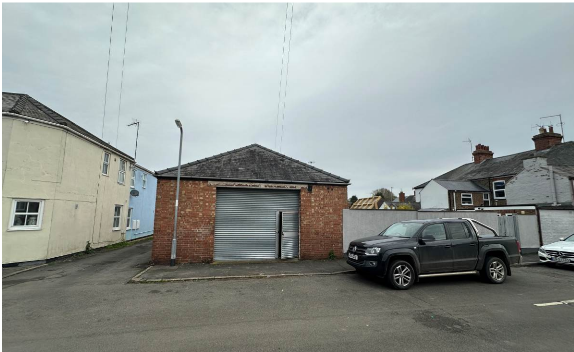
Front view of existing building from King Street
