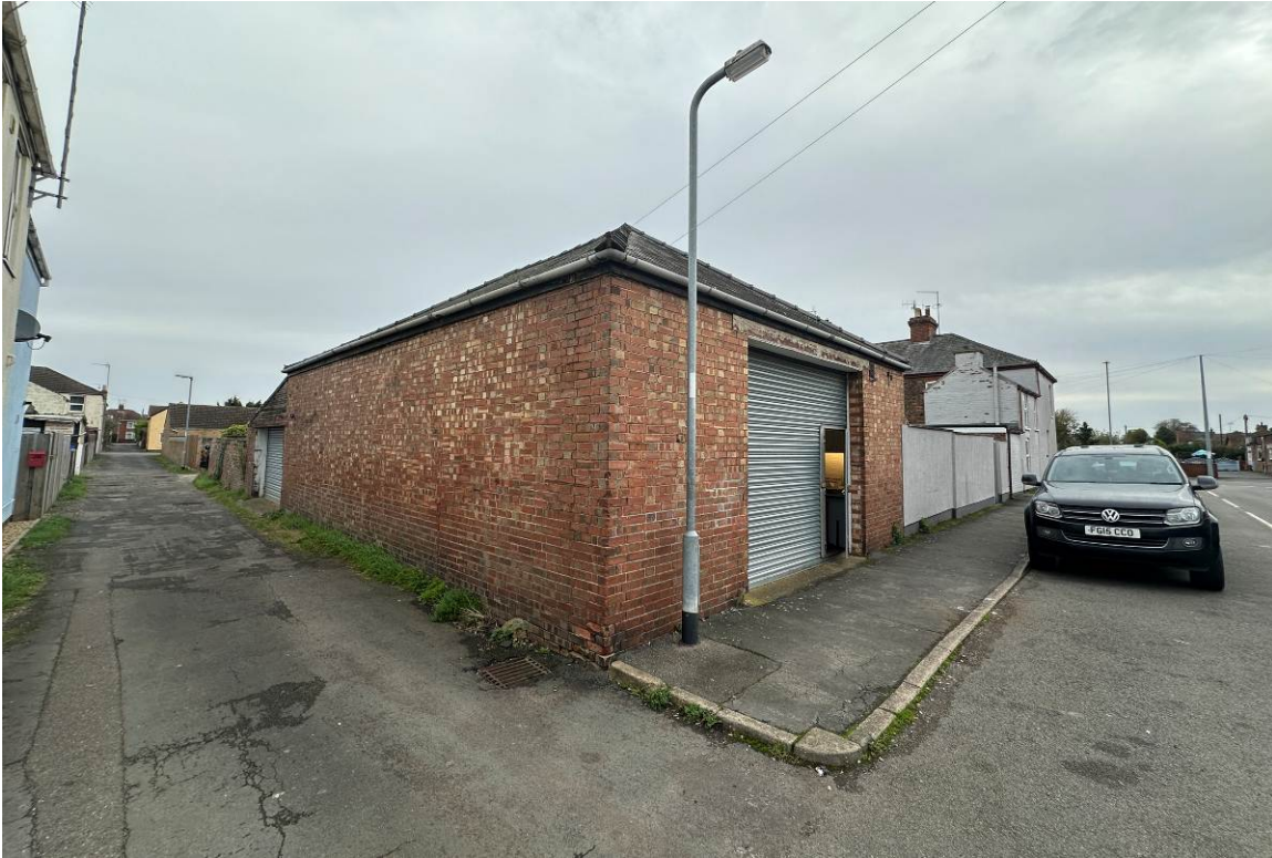
Front/Side view of existing building from King Street
