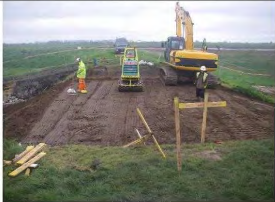
Compaction and testing of 3 rd reinstatement layer (looking west).
