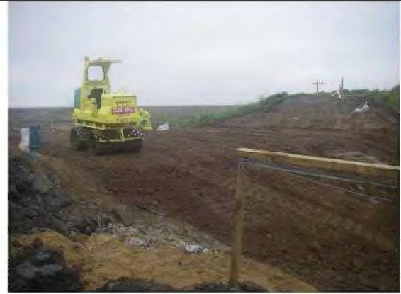
Compaction of 1 st reinstatement layer through breach (looking east) and nuclear
