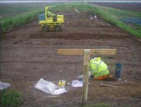
Testing and compaction of 2 nd and 3 rd reinstatement layers (looking
