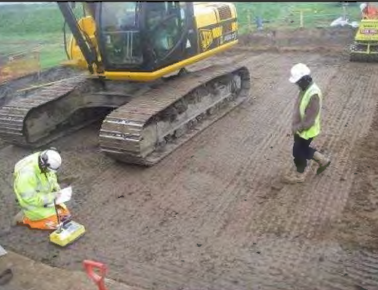
Compaction and testing of 4 th reinstatement layer (looking west).
