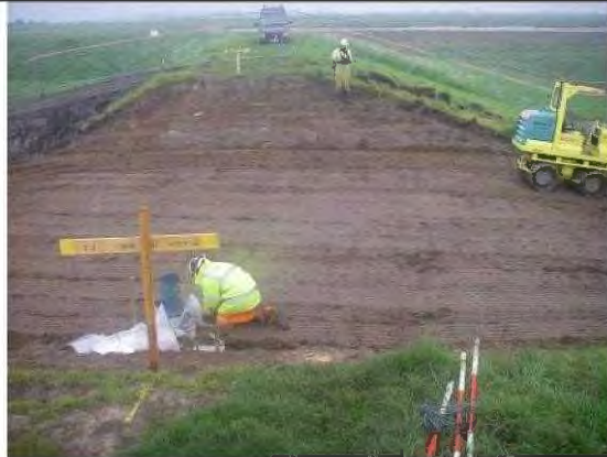
Compaction of 1 st reinstatement layer through breach (looking west) and sand replacement
