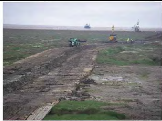
Retrieval of 100mm bogmat units. Trencher/cable layer Nessie III at the seaward edge of the saltmarsh.
