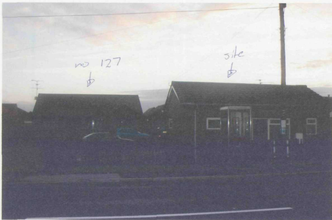
view south from road
