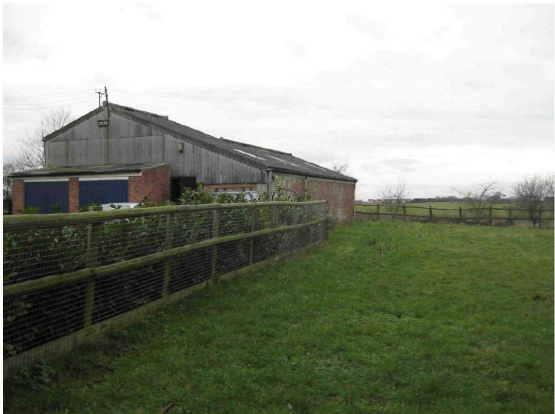
Figure 7: North Easterly View of the Existing Barn to be Demolished
