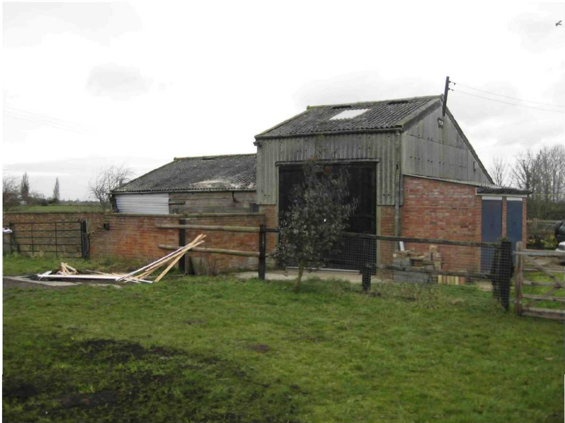
Figure 6: Southern View of the Existing Barn to be Demolished
