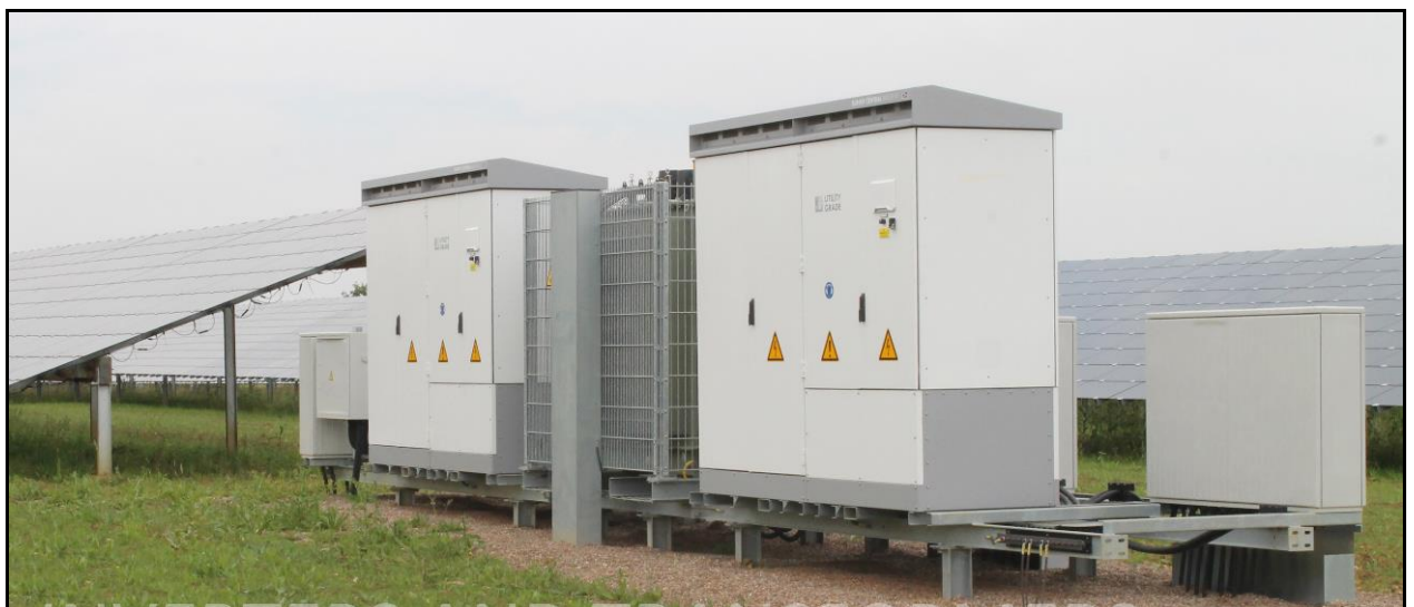
Figure 6c – Inverter and Sub-station Switchgear
