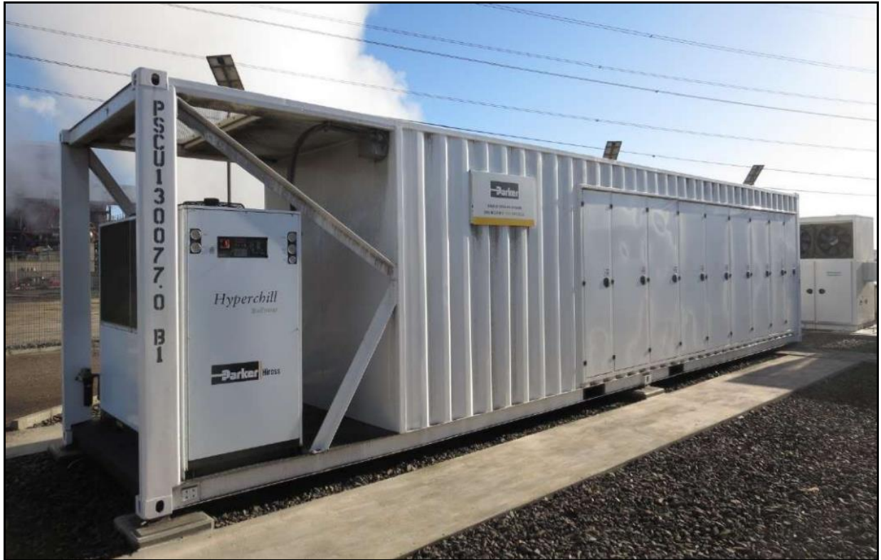
Figure 6d – Battery Storage Units
